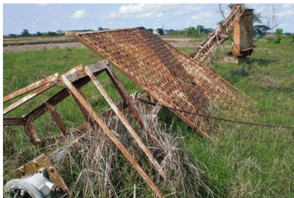
Photo 4.2.9 Damaged Back Leading Light at Thanlyin Point ④
