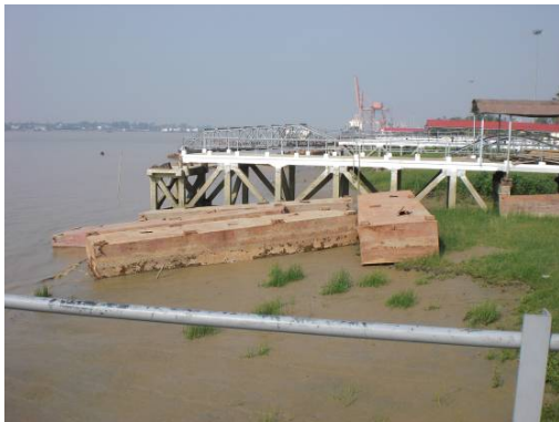
Source: JICA Project Team
