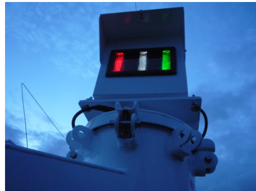
Monkey Point Sector Light Properly Working at Night Time
