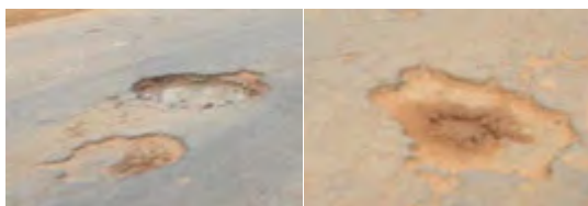
Figure 1.1 Potholes
