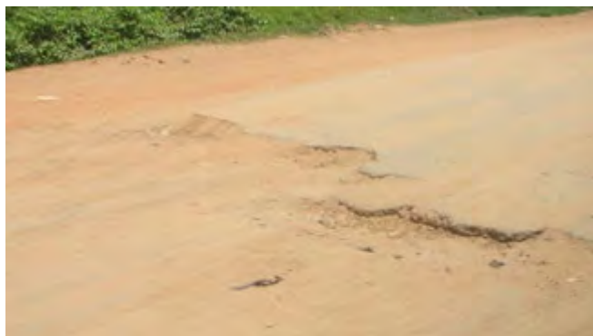
Figure 1.2 Pavement Failure
