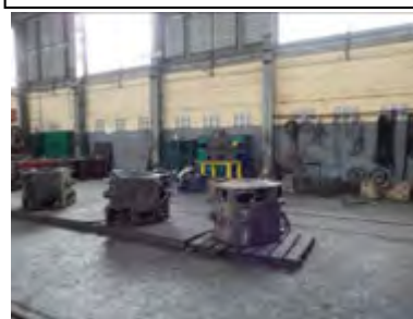
Inspection of electric generators
