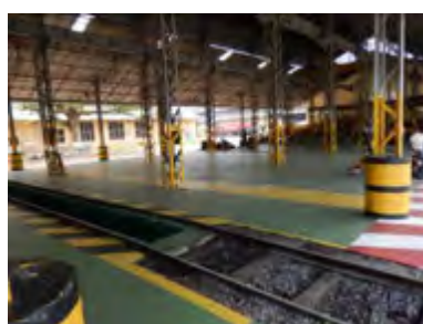
Track maintenance equipment area & shed
