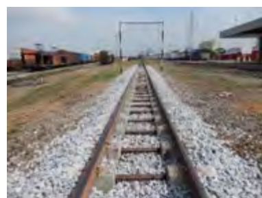
Inspection track after Ballast maintenance
