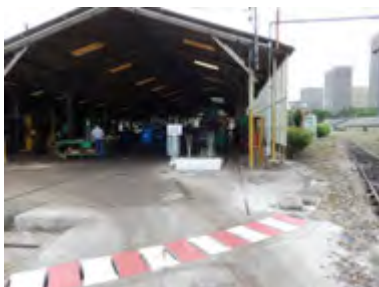
Wheel maintenance and repair shop.
