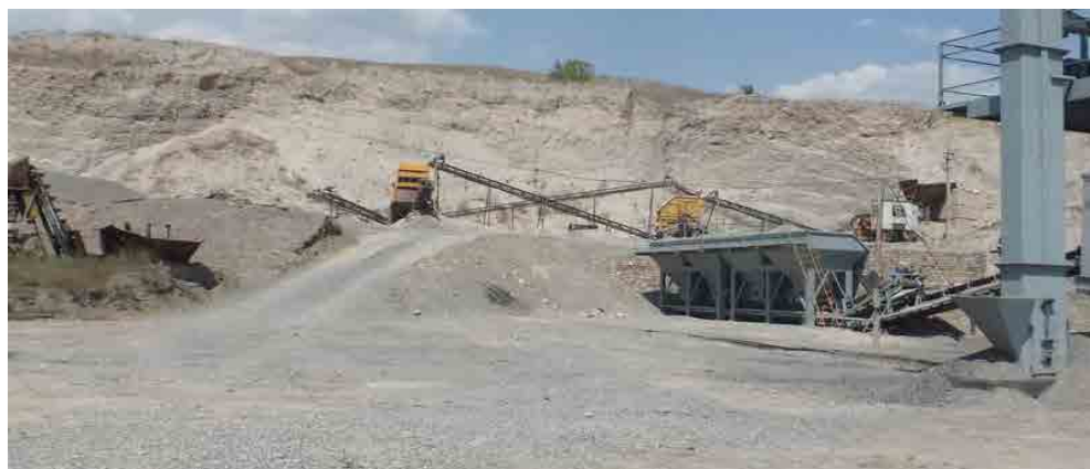
Quarry Site No. 1
