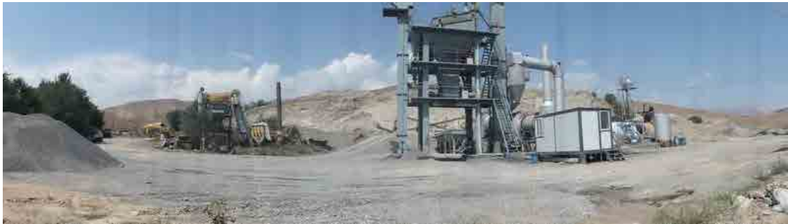
General View of the Asphalt Plant for the Project
