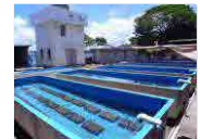
Sea water aquafarming facility (introduced in Phase 1)
