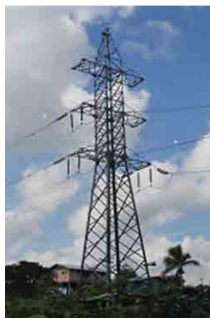
Figure 6.10.4-2 132kV D/C Designed Tower Near the Cunningham Substation Under S/C Operation
