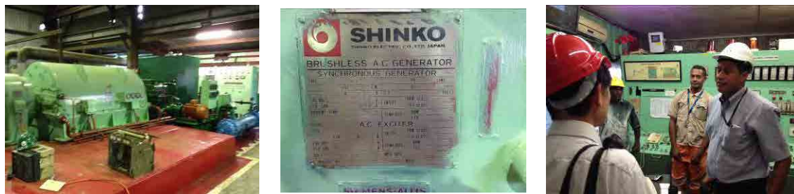
Turbine and Generator (SHINKO; JAPAN)
