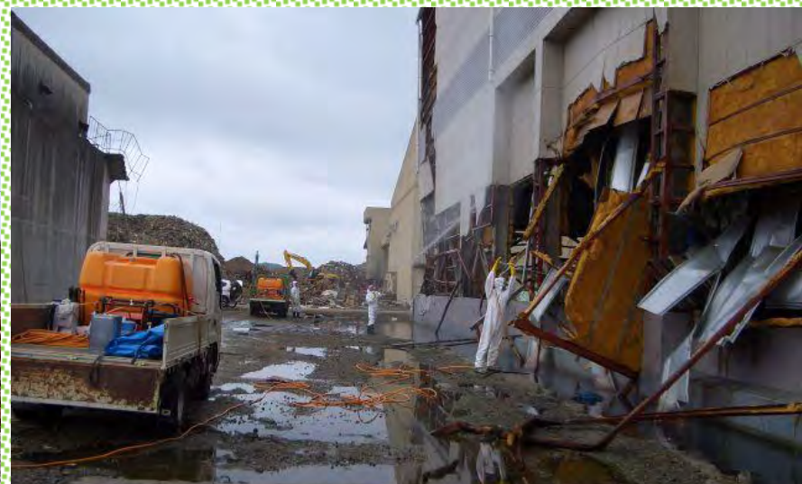
Spraying to rubble heaps and broken freezer by PC operators
