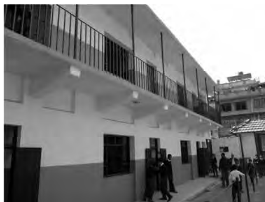
Adarsha Higher Secondary School (耐震補強後の校舎)
