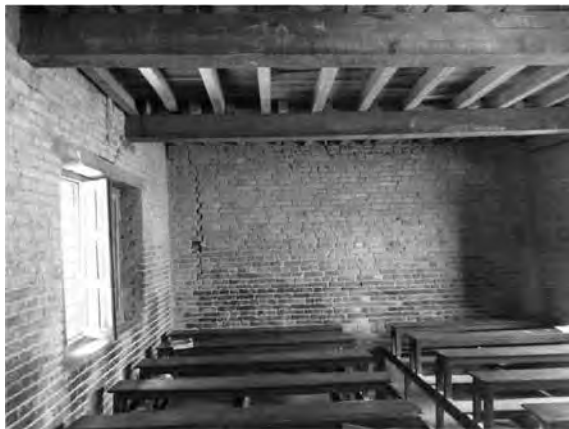
Ganesh Secondary School (補強前の教室、2階の梁と床は木造)
