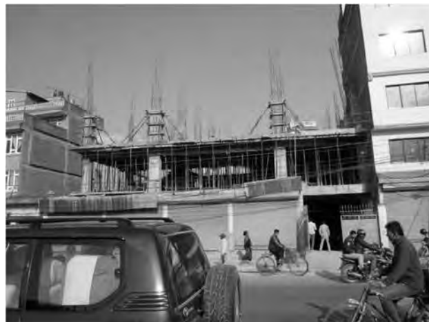
Construction Site in Relatively New Town (Old Dhalku)
