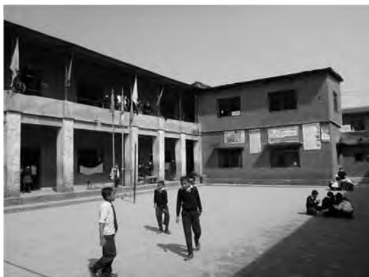
Adarsha Higher Secondary School (補強前の校舎)
