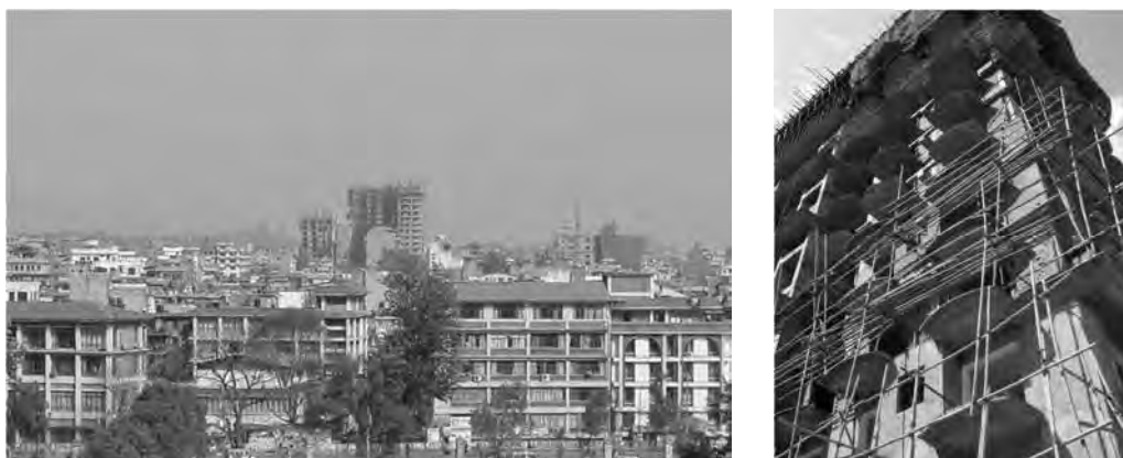
Photograph 2 One Sample of High-Rise Building Construction
