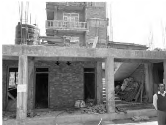
Ganesh Secondary School (新築中の校舎)
