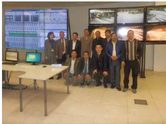
Observation of control room of Hai Van Tunnel
