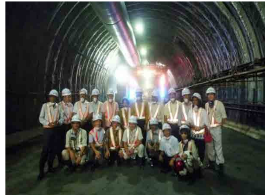
Observation of Tarutouge Tunnel Construction Site
