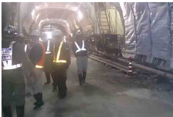
Observation of On-going Construction Work Inside Shimoshiobara 2 nd Tunnel
