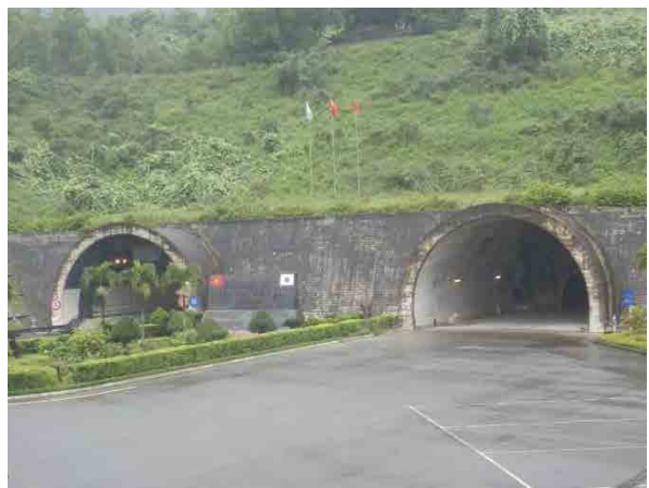
Observation of Hai Van Tunnel in Da Nang
