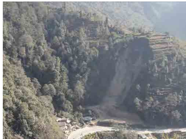
FIGURE 6.2-8 LARGE LANDSLIDE NORTH OF THE SISNE KHOLA
