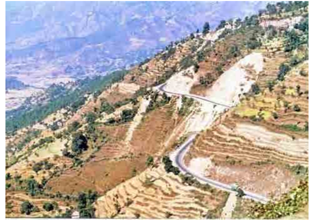
FIGURE 6.2-10 CUTSLOPE COLLAPSE AFTER HARD RAINFALL
