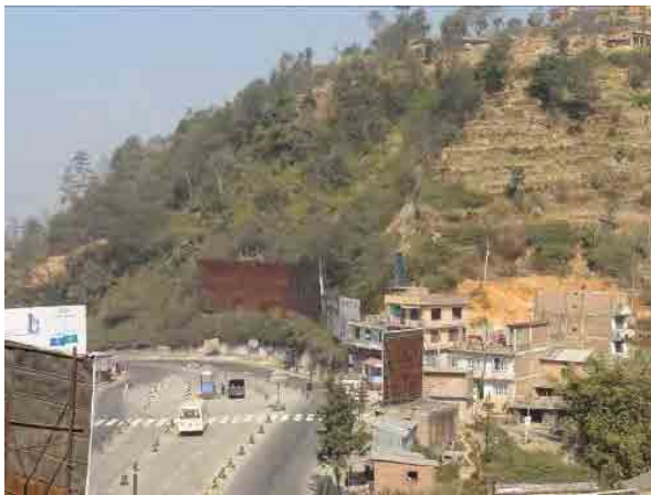
FIGURE 6.2-7 LARGE LANDSLIDE NORTH OF CHECK POST
