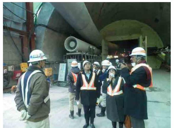
Observation of On-going Construction Work of Tarutouge Tunnel
