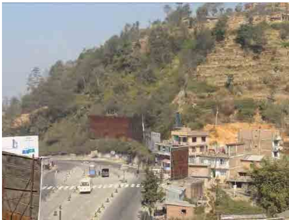
FIGURE 6.2-7 LARGE LANDSLIDE NORTH OF CHECK POST
