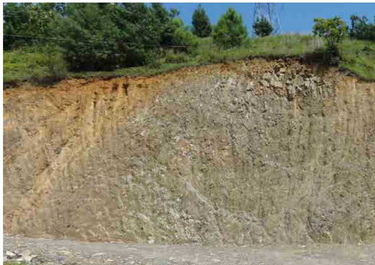
FIGURE 4.2-13 FAULT WITH FRACTURED ZONE
