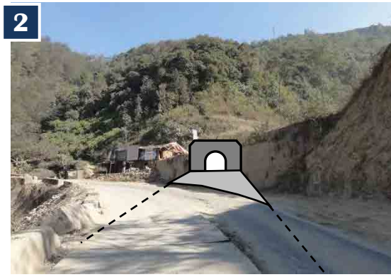
Image of West Side Tunnel Portal (Naubise side)
