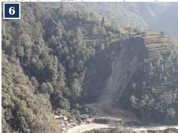
Recent slope failure near objective road
