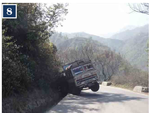
Traffics (Trucks) are frequently found stuck in open drainage
