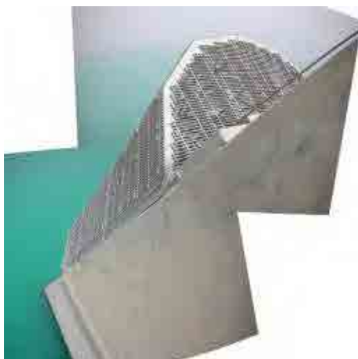
Fig. 3.6-4 Trashrack of Jazira Intake
