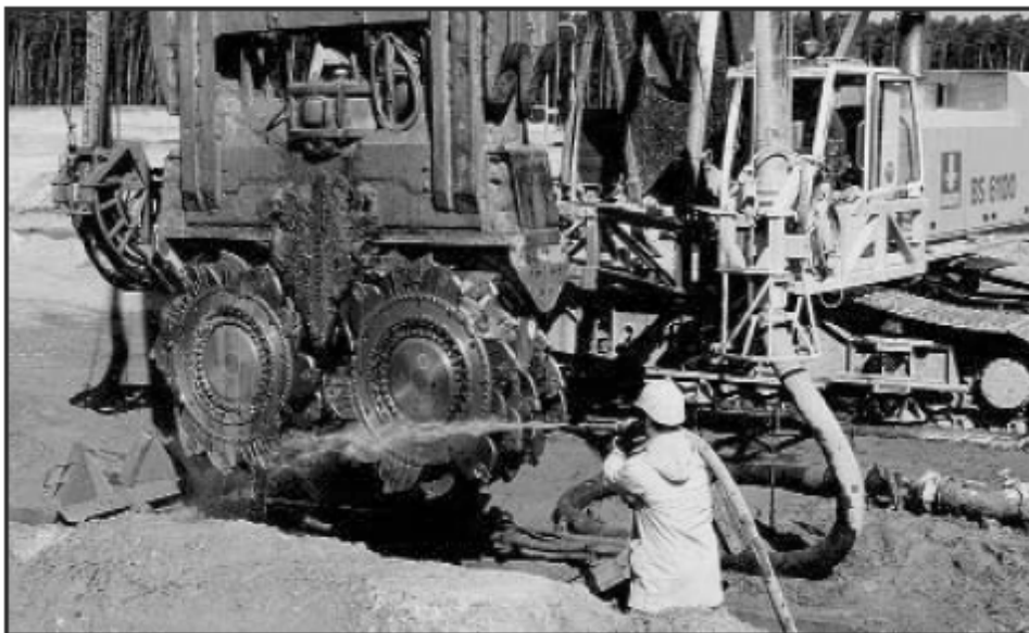
Fig. 3.6-13 “Hydromill Type” Equipment for Diaphragm Construction
