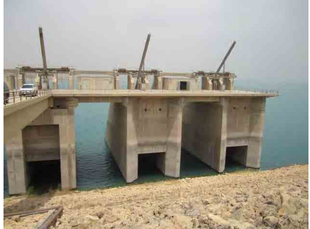
Intake structure for Hydraulic Power Plant at Mosul dam
