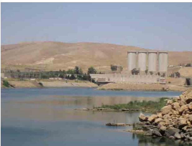
A view for the Mosul Hydraulic Power Plant at Mosul dam
