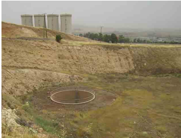
Bypass shaft, starting point of feeder canal at Mosul dam
