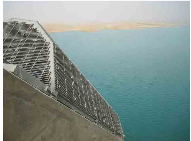
Screen of the intake for the Suoth Jazira Irrigation Project, Mosul dam
