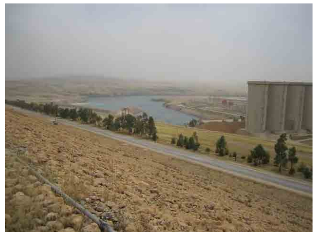
A view of Mosul dam downstream, Tigris River
