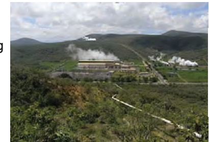
Geothermal Power Plant
