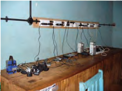
Power outlets on the wall and a shelf are convenient for the operation.
