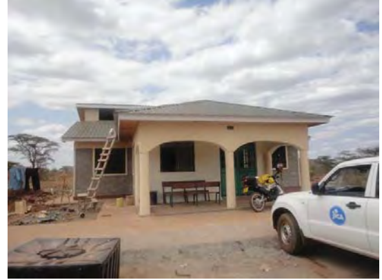
Photo 1.2 Main Dispensary Building
