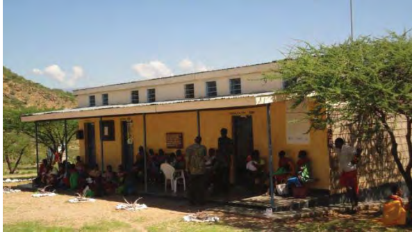
Photo 4.1 Main Dispensary Building
