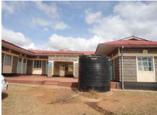
Photo 2.1 Meto Dispensary Building
