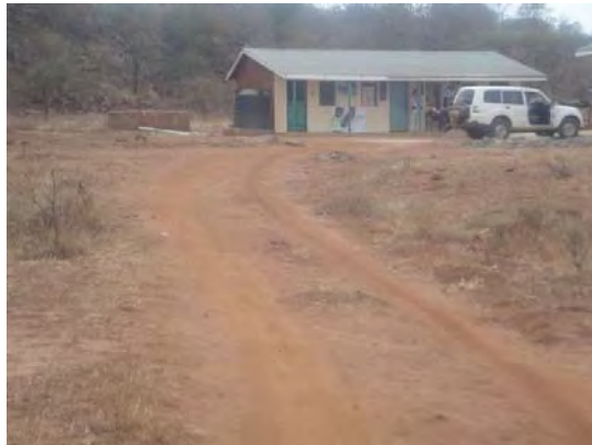
Photo 1.3 Access road to the Dispensary
