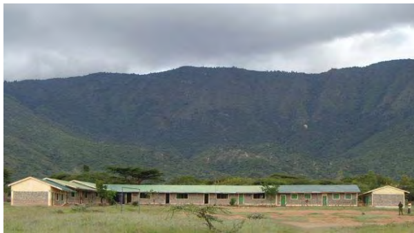
Photo 1.5 Surrounding Land Features
