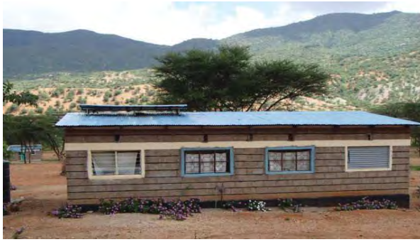
Photo 5.1 Main Dispensary Building (Back Side )
