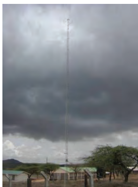
Figure 1 Wind Monitoring Station in Baragoi
