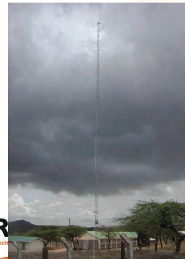
Monitoring Height: 20m, 40m Anemometer, Wind vane
