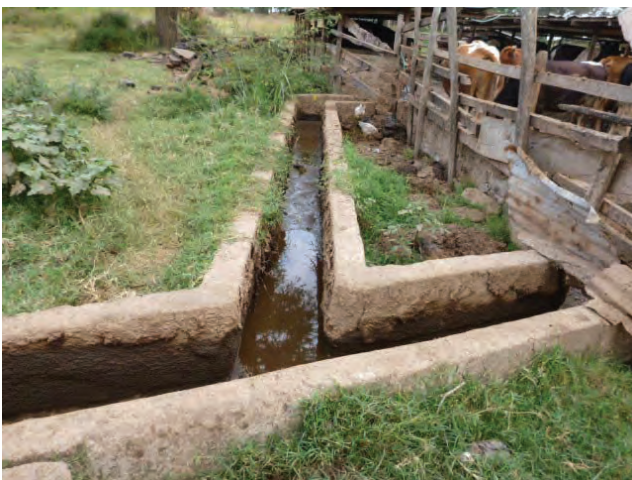
Ditch for cow dung and waste connected to digester
