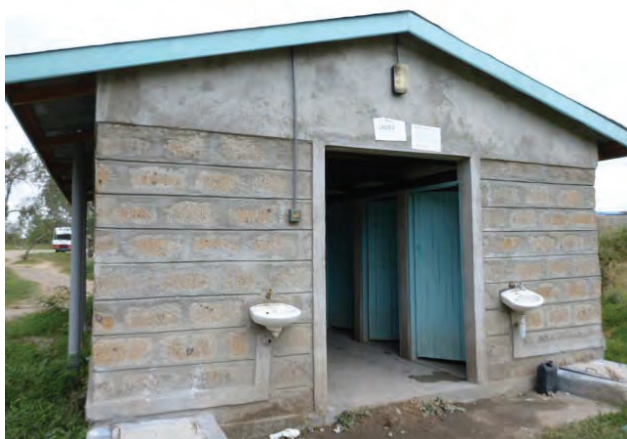
Toilet to supply human waste to digester
