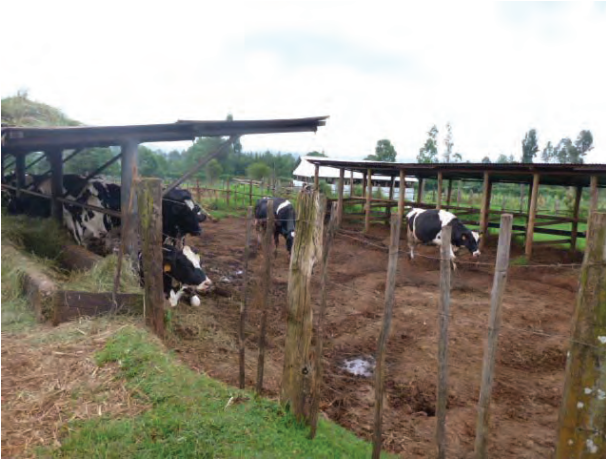
Cow shed, need floor cement placement
