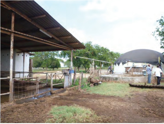
Cow shed, collection chamber, and biogas dome
