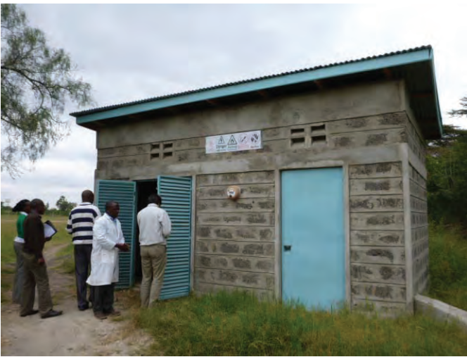
Power House for Genset and Gas Holder
