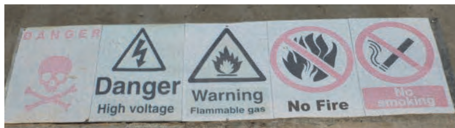
Photo Fire Extinguisher and Warning Sign
