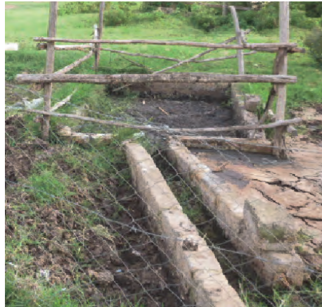
Figure 2.2.2 Open Ditch and Connection to Feeding Chamber
