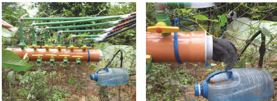
Photos Steel Wool Type Biogas Filter
