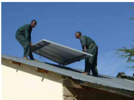
Installation Work (PV 1) Illaut Primary School
