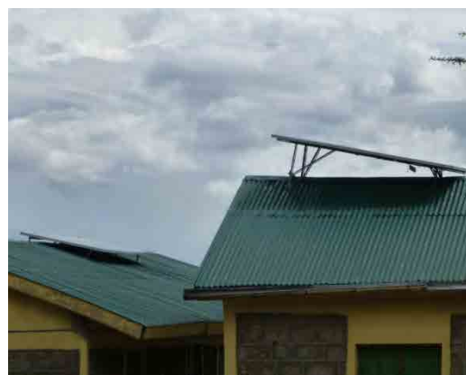
Installations of PV Array (Tuum Pry. School) (facing North)
