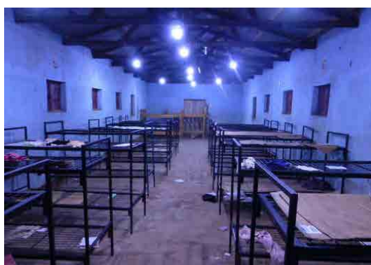
Dormitory with Installed Lights
