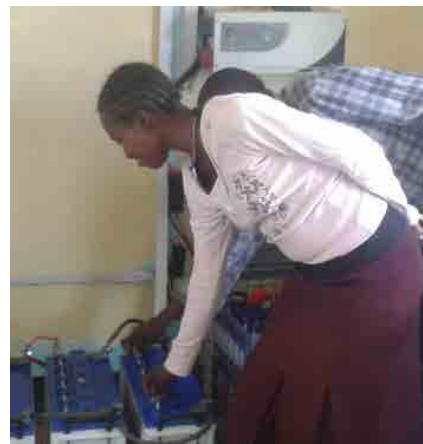
Measurement of Battery after Replacement
