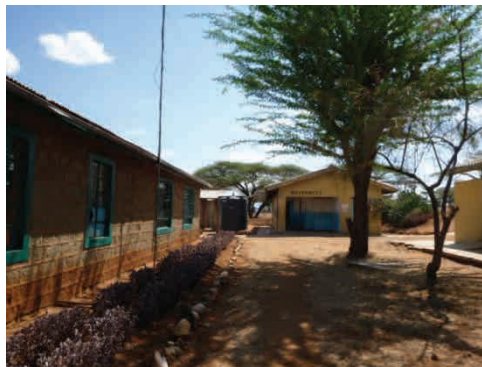
Baragoi District Health Office
