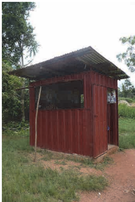
Charging station is not so large.
