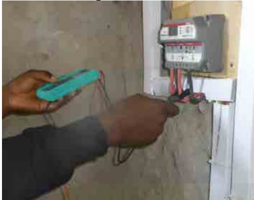
Measurement of CC after Replacement
