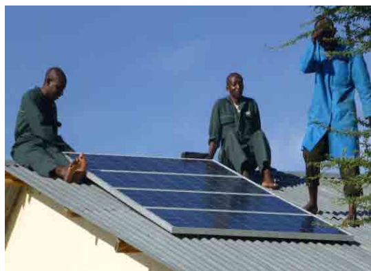
Installation Works (PV 2) Illaut Primary School
