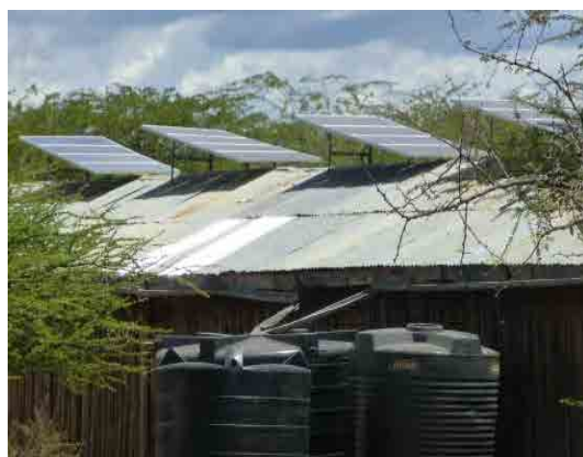
PV Array for Computer System (DC 48 V) At Marti Pry. School (facing North)
