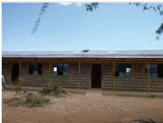
Marty School Classroom and existing PV Panel
