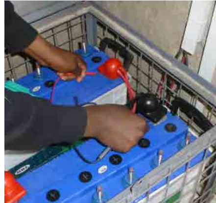
Measurement of Battery after Replacement
