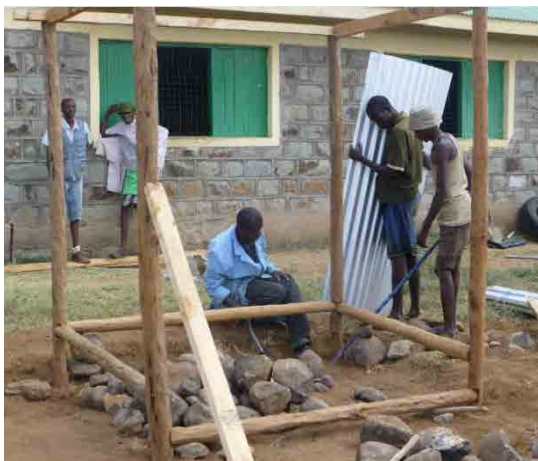
Construction of Charging House
