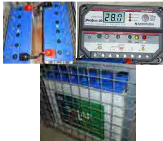
Newly Replaced CC and Battery
