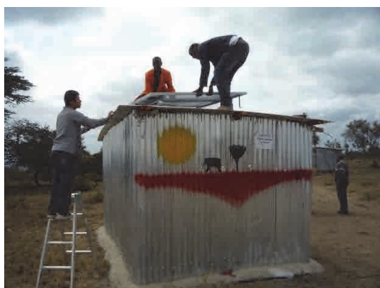
Photo 3 Installation of Charging System
