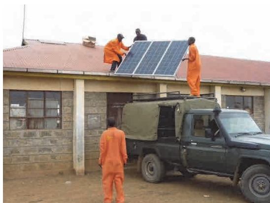
Photo 1 Installation of Solar Panels
