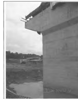
Viaduct 1 Pier No.2 at A1 Bypass
