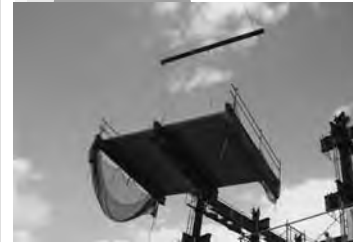
Lifting and installation work
