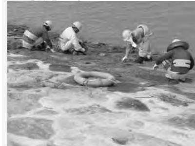
Workers are wearing Ski Belt while working on the slope
