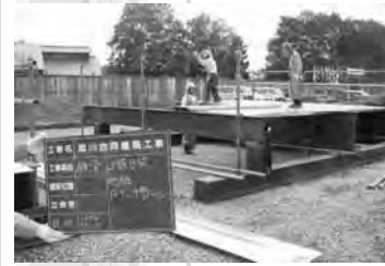
Work on ground
