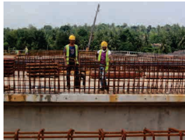
Chipping Construction Joint
