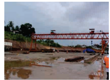
Girder Fabrication Yard (N)
