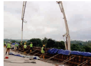
Parapet Concreting (1)
