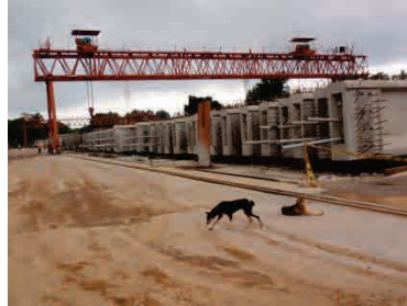
Girder Fabrication Yard (S)
