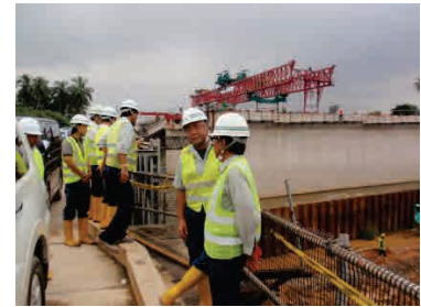
Temp. Bridge on Kelani River
