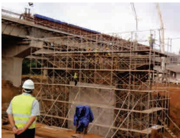
Scaffolding for Ramp Pier
