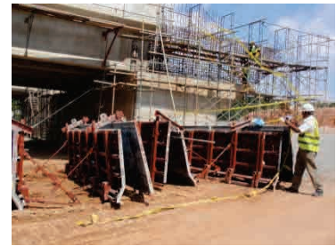
Parapet Formwork
