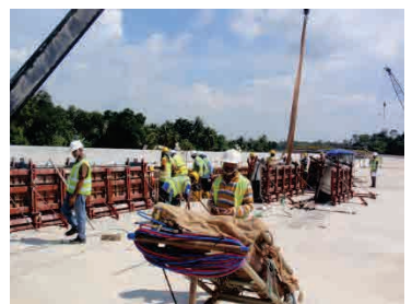
Parapet Construction
