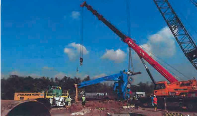
The crane removing operation
