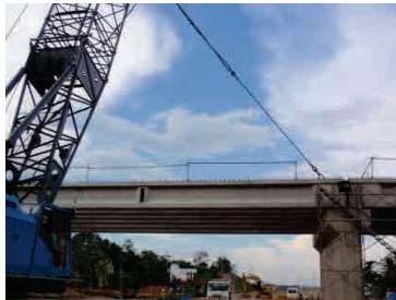
Erection of PC Girder
