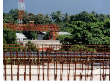
Girder Fabrication Yard
