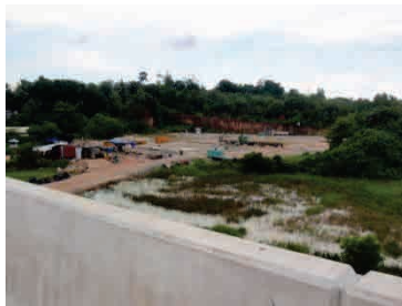
PC Girders Temp. Storage Yard
