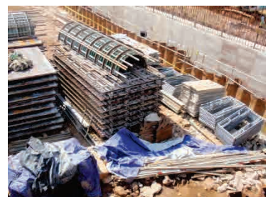
Formwork Storage at Kelani River
