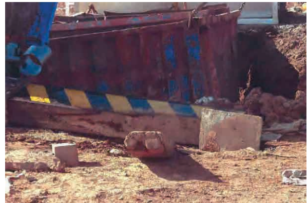
The outrigger arrangement (Timbers were used.)
