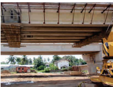
Scaffolding supported by brackets
