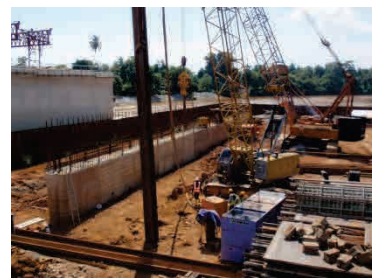
Extracting Sheetpile at Kelani River
