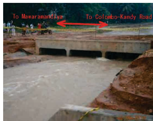
The box culvert under construction
