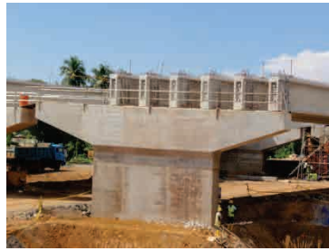
PC Girders & Pier
