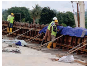
Parapet Formwork
