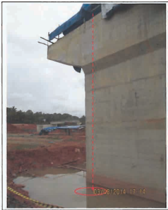
Viaduct 1 Pier No.2 at A1 Bypass
