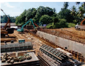
Pier Construction at Kelani River
