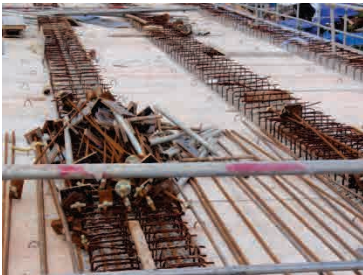
RC Slab Soffit Form
