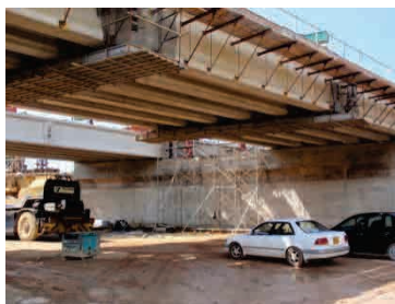
Scaffolding supported by brackets
