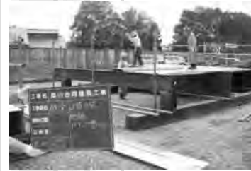
Work on ground
