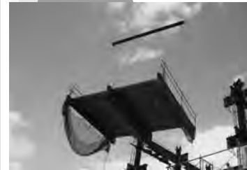
Lifting and installation work
