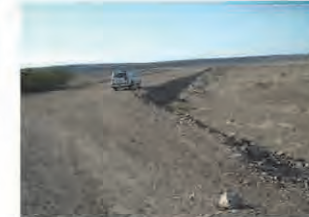
Access road is completed
