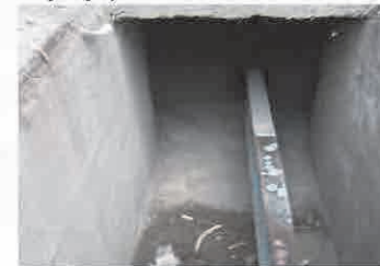
Inside of the pit is kept dry
