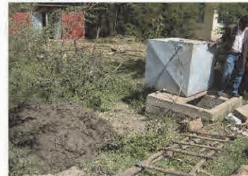
Well point and mud removed from ditch
