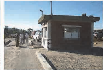
Weighbridge and control house
