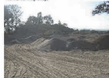
Off loading site
