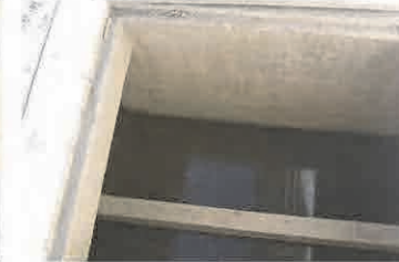
Water filled in the pit
