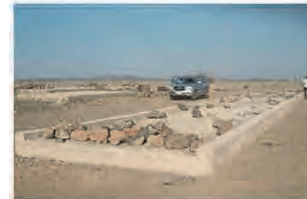
A pit for an axle load scale is under construction (4m x 37m). The scale shall be one axle load scale. Foundation for Control Room and Office are completed
