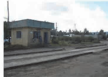
Truck scale and control house
