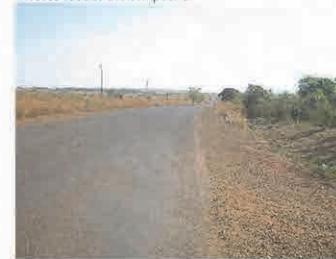
Road and access road
