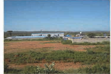
Compound of road construction company (ERA's property)
