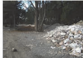
Off loading site
