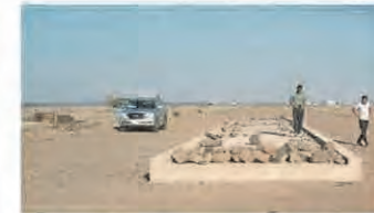
A pit for an axle load scale is under construction (4m x 37m). The scale shall be one axle load scale. Foundation for Control Room and Office are completed
