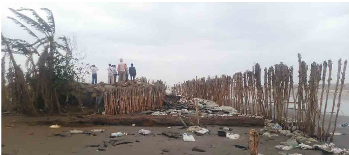
Photo 2.1.1 Current beach conditions about 1 km north of the Duyen Hai CFPP (wooden piles seemingly for beach erosion protection are placed in front of the house. Photo by the JICA Study Team)
