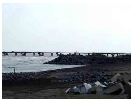
Photo 2.4.2. East Breakwater and Trestle for Coal Transshipment (March 2014 by the JICA Study Team)
