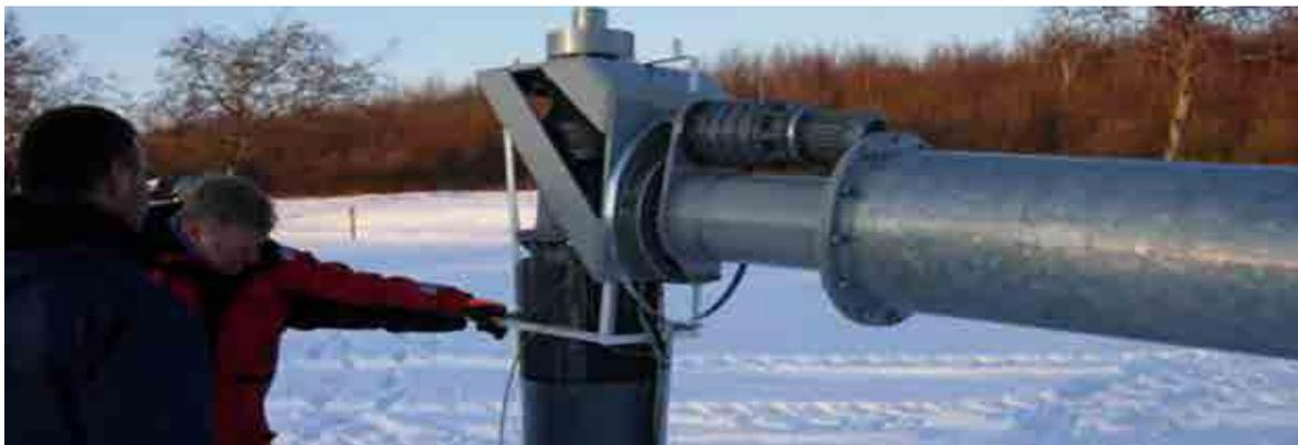
Since the heaviest lifting when installing the turbine is of the 750 kg nacelle to a height of 2 meters, no crane is necessary. A tractor or the like can easily be used to fit the nacelle.
