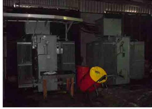
Feeder pressure transformer(13,800/480V)
