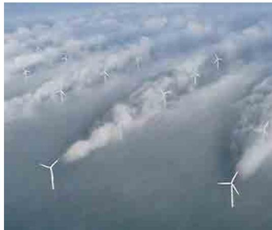
Figure 3.3.3-3 Effect of wind turbine separation
