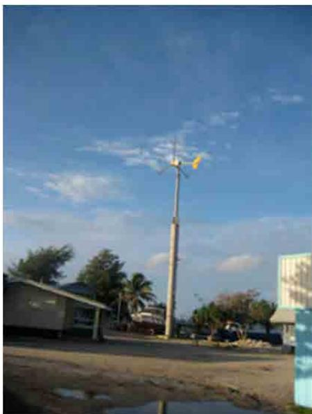
Figure 2.3.2-1 RRE 7kW wind turbine
