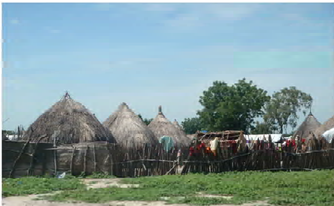
“Tukuls” are traditionally made by “gottiya sticks” with a straw thatched roof. More tukuls are seen in the Eastern and Southern Payam.
