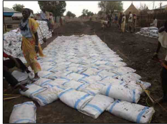
Photo 22.1-1 Actual Diagonal Herringbone Layout
