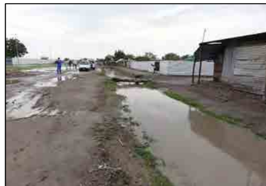
Storm Water Drainage (Main Drain)
