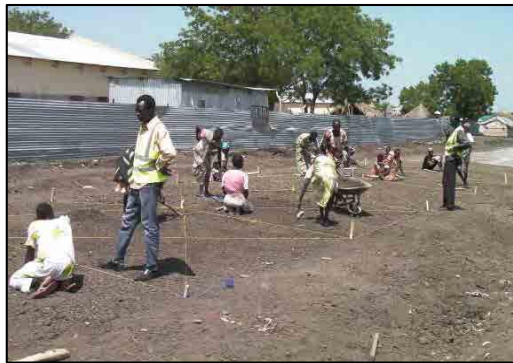
Construction Work by Labour Based Technology (LBT)
