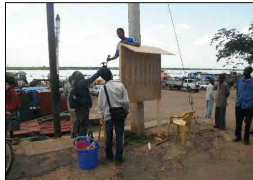
Installation of Project Signboard
