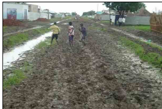
Community roads easily get muddy in rainy season. LBT Construction Site (Upper Part)
