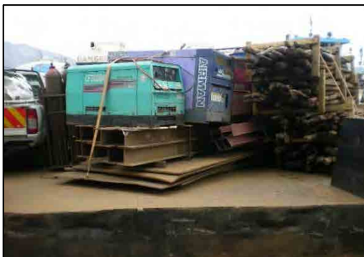
Loading Construction Materials at Juba River Port
