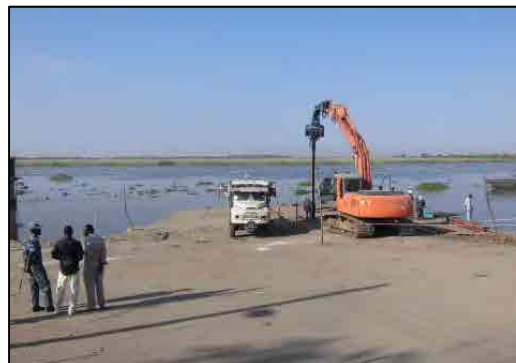
Piling for Reinforcement of Existing Jetty
