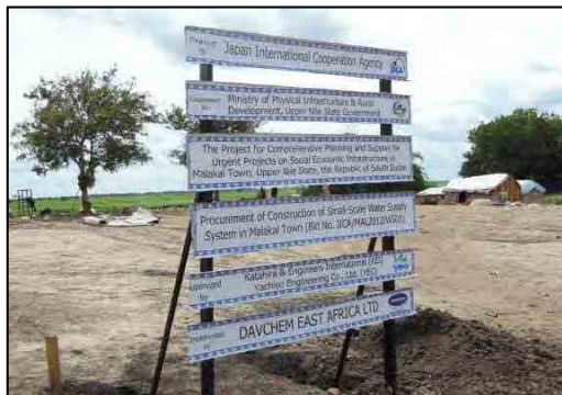
Installation of Project Signboard
