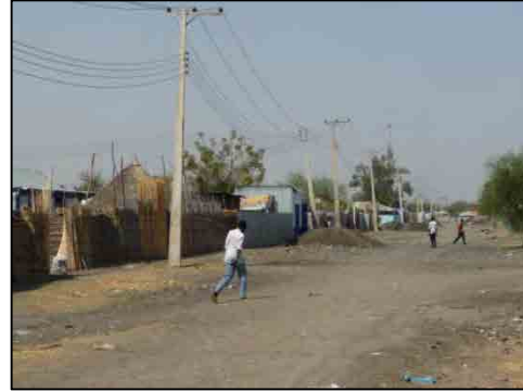
11kV & low voltage (LV) Line
