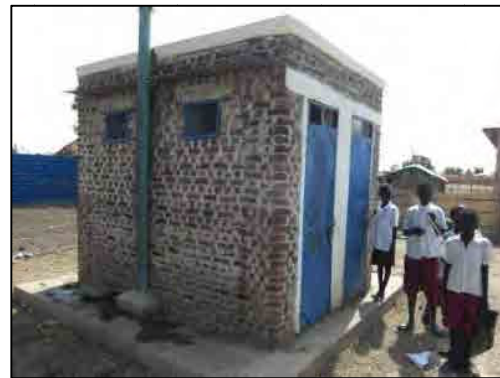
Primary School Toilet in Assossa
