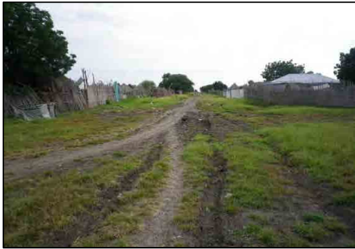
Condition of Existing Community Roads in Malakal Town
