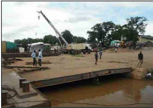
Present Situation of Cargo Jetty Before Construction
