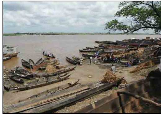
Present Situation of Passenger Jetty Before Construction
