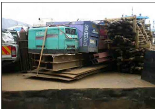
Loading Construction Materials at Juba River Port
