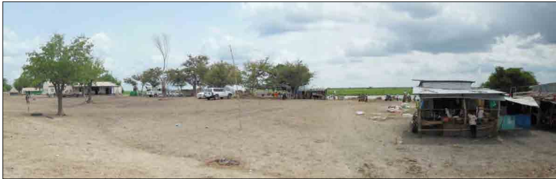
Construction Site of Water Treatment Plant Before Construction
