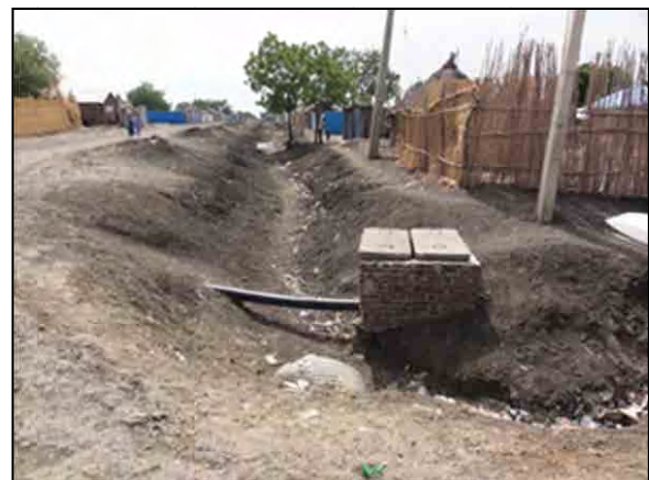
Photo A Main Drain in Malakal Town
