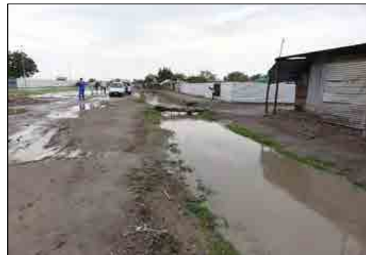
Storm Water Drainage (Main Drain)
