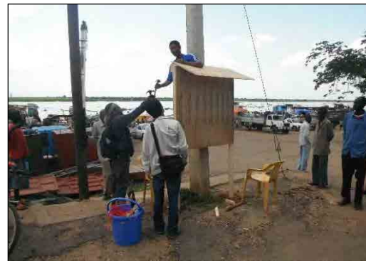
Installation of Project Signboard
