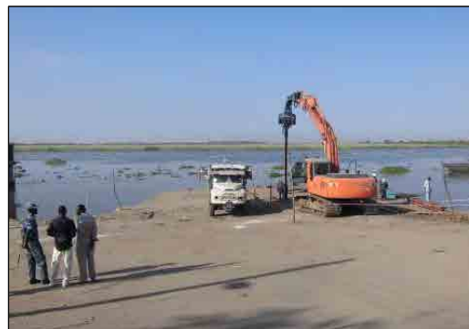
Piling for Reinforcement of Existing Jetty
