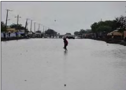
Photo: JICA Project Team Road Inundated in Rainy Season
