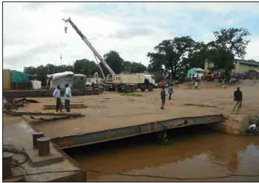
Present Situation of Cargo Jetty Before Construction
