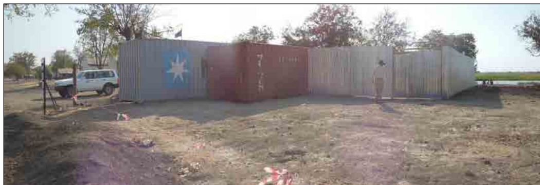
After Leveling of the Ground, Removal of the Facilities and Storage of the Equipemnt and Construction Materials
