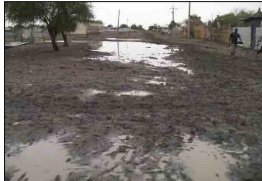
Decreased Traffic Performance due to Mud
