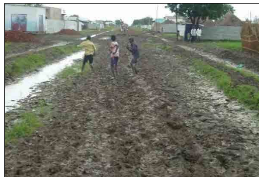
Community roads easily get muddy in rainy season. LBT Construction Site (Upper Part)
