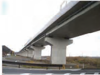
• PC pretension slab bridge
