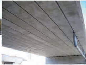
• PC posttension hollow slab bridge
