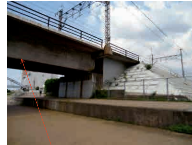
Prestressed concrete girder(5spans)
