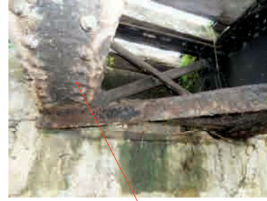
Corrosion
