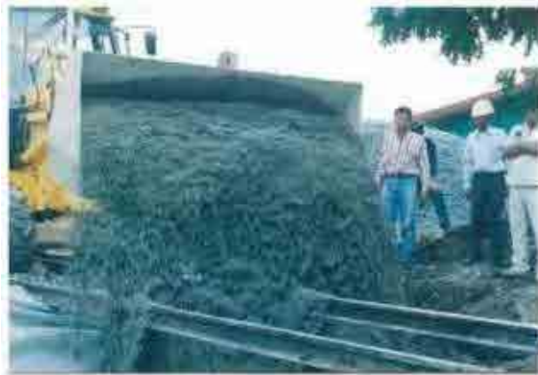
In the rehabilitation work of Thai railways, sand was used as the sub ballast
