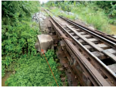
Collapsed abutment
