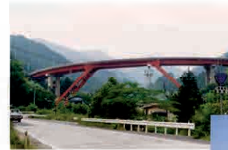
• Steel rigid frame bridge
