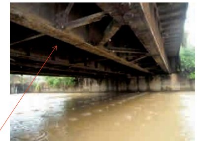
Corrosion
