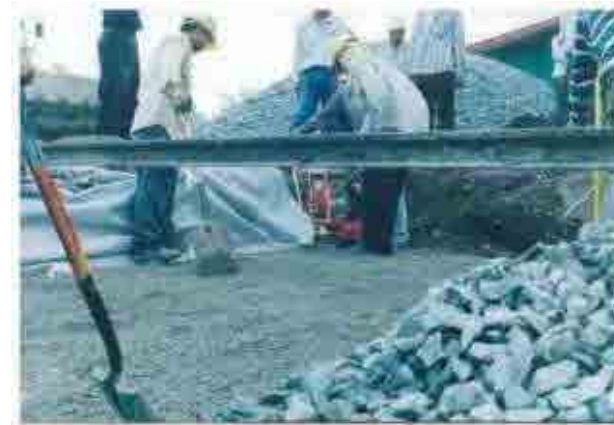
Sand was leveled and tamped by vibration equipment. Water stopping sheet was spread under the sand.(Example of Thai railways' rehabilitation works )
