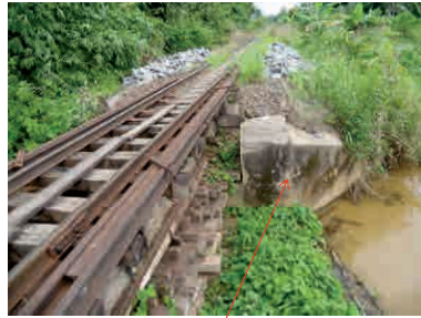
Collapsed abutment
