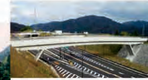
• PC \pi style rigid frame bridge
