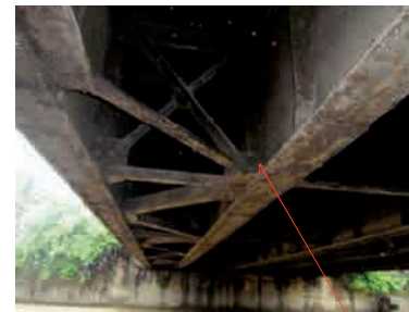
Corrosion
