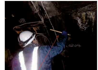
Inspection of float by hammer
