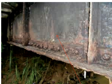
Corrosion
