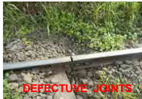
DEFECTIVE JOINTS
