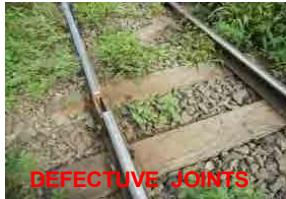
DEFECTIVE JOINTS
