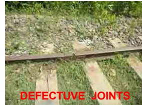
DEFECTIVE JOINTS
