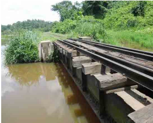
(a) Steel Upper-Deck Plate Girder
