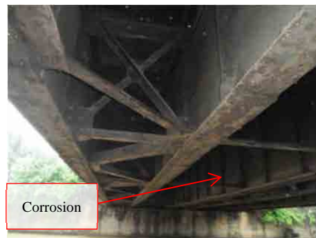
Photo 4.2.32 Steel Beam of Busua Bridge
