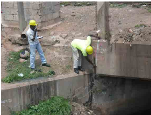
Photo 4.2.16 Measurement of Beam Height
