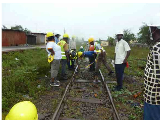
Photo 4.2.72 The Trainees are measuring the track irregularity after finishing the maintenance work
