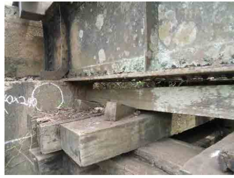
Photo 4.2.41 The state of the sleeper were piled up don't support upper structure (2)
