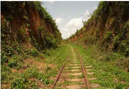
(d) Cut section (laterite soil cut and left as is)
