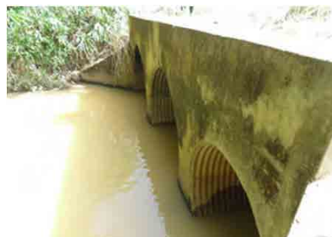
(c) Pipe Culvert (Armco Pipe)
