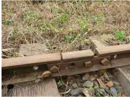
Photo 2.3.45 Extremely Short Rail in the Joint Gap (Dunkwa - Awaso)
