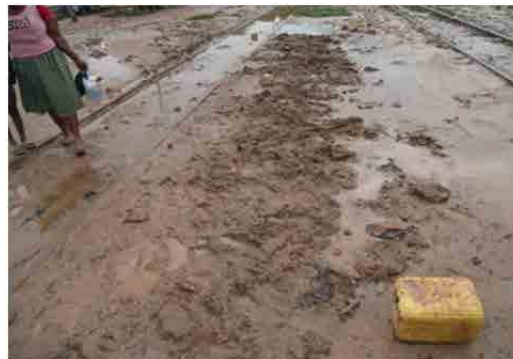
Photo 2.3.33 Water and Soil Flowed onto the Track in Kojokrom Station
