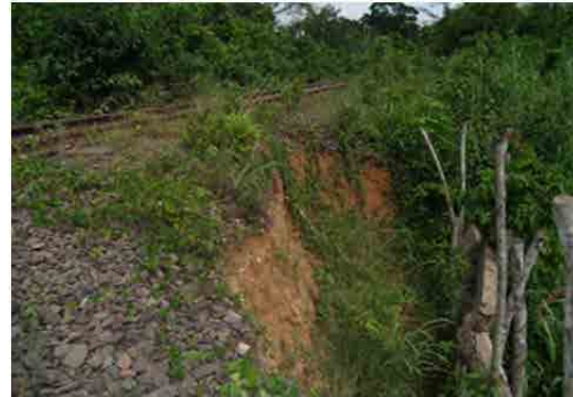
(c) Embankment Collapse on the Track Side
