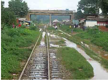
Photo 2.2.7 Station Yard in which Effluent Flows through the Track Areas like a River (Kojokrom Station area on the Western Line)
