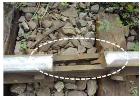
Photo 2.3.44 Broken Rail End at the Joint (Kojokrom - Angu)
