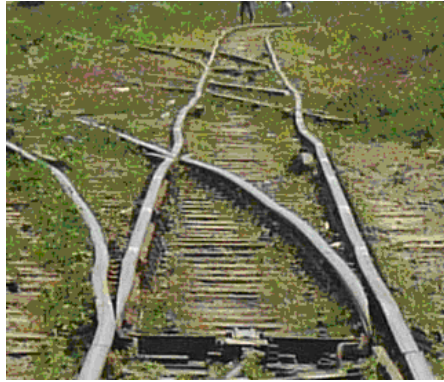
Photo 4.2.56 There are many big track irregularity spots (Butuah St. Yard)
