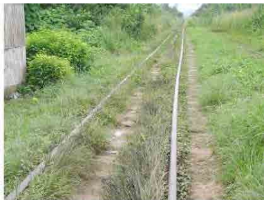
Figure 4 Waving Track
