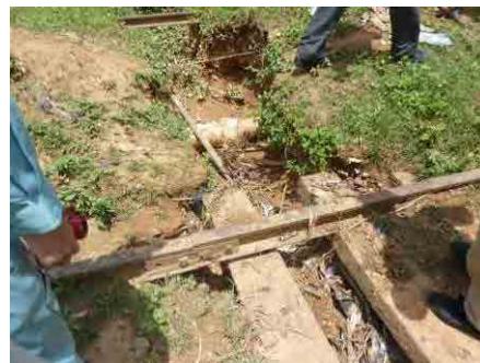
Photo 2.2.10 Ballast and Roadbed Eroded by Water Flowing from a Residential Area (Maudaso-Ankwaso on the Awaso Branch line)
