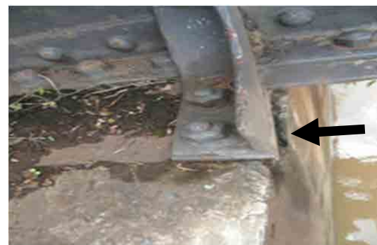
(d) Concrete Spalling at the Face of Bridge Seat (Bridge No.1)
