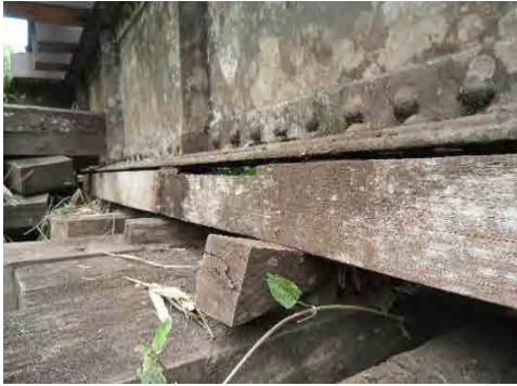
Photo 4.2.40 The state of the sleeper were piled up don't support upper structure (1)
