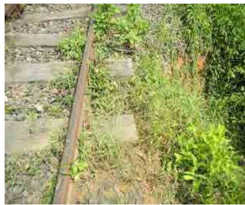
Photo 2.3.14 Collapsed Roadbed (2)
