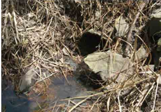
(b) Culvert Covered with the Sediment
