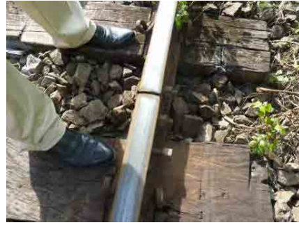
Photo 2.3.46 Lack of Fish Bolt and Loosening Nut (Kojokrom - Angu)
