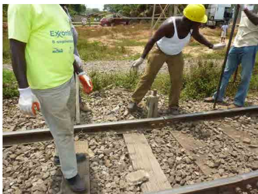
Photo 4.2.68 The Trainees are lifting the low joint by the track jack
