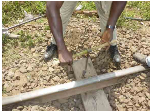
Photo 4.2.65 Trainee is drilling the hole into the sleeper by auger
