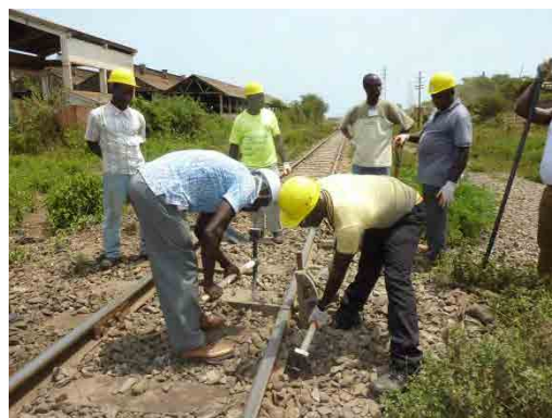
Photo 4.2.69 The Trainees are tamping the ballast under the sleeper
