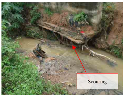
Photo 4.2.37 Retaining Wall Foundation be Scoured in Ghana
