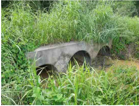
Photo 2.3.35 Diverted River and New Culvert
