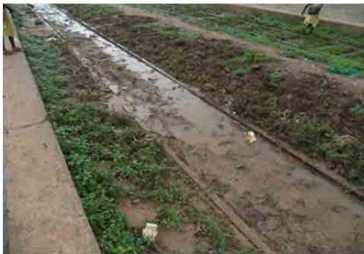
Photo 2.3.33 Water and Soil Flowed onto the Track in Kojokrom Station
