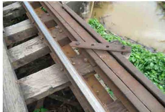
Photo 2.3.36 Track Protection by Rail Girder
