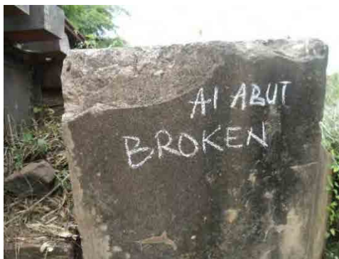
Photo 4.2.42 The State of the Collapsed A1 abutment (1)
