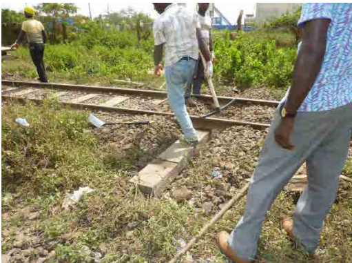
Photo 4.2.64 Trainees are inserting the used sleeper
