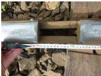
Photo 2.3.43 Excessive Joint Gap beyond 130mm (Kojokrom - Angu)
