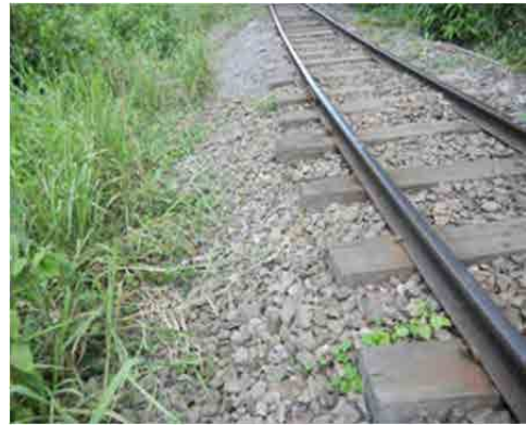
Photo 2.3.8 Ballast beside Sleepers
