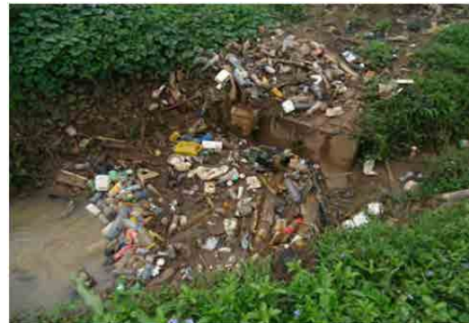
Photo 2.3.32 Culvert Filled with Garbage in Kojokrom Station
