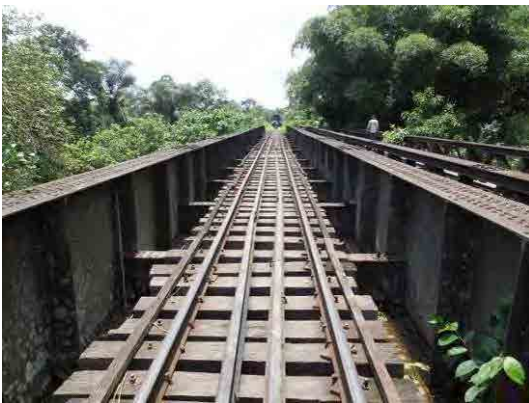
(b) Steel Through Plate Girder and Steel Through Truss Girder
