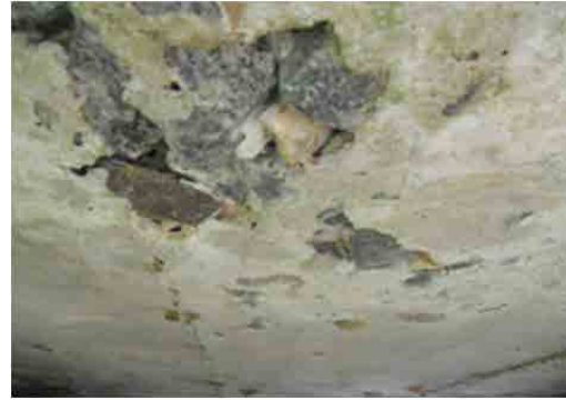
(a) Spalling of the Concrete
