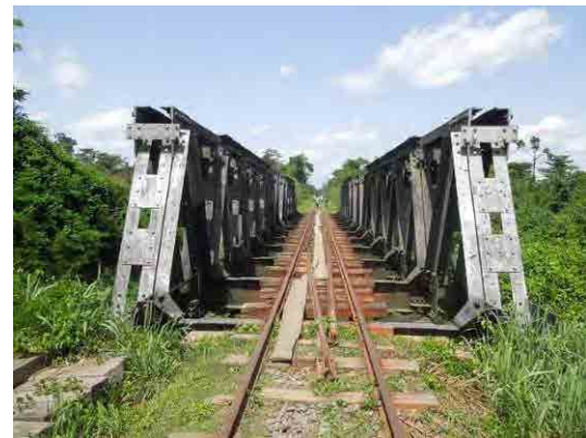
(b) Steel Through Plate Girder and Steel Through Truss Girder
