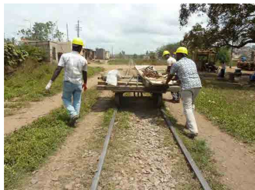
Photo 4.2.67 The Trainees are transporting the sleeper on the trolley.
