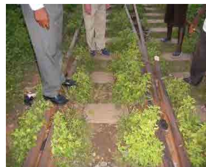
Photo 10 Trace of derailment (Dunkwa)
