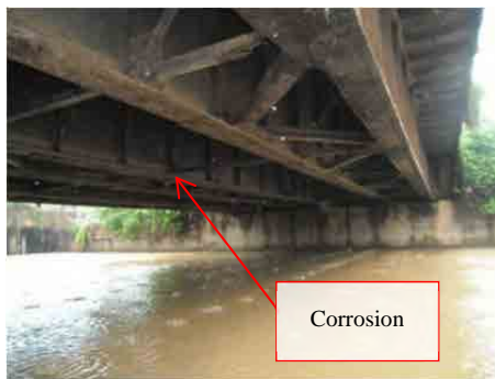
Photo 4.2.31 Steel Beam of Busua Bridge
