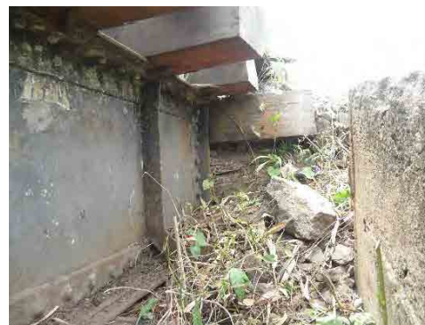
Photo 4.2.43 The State of the Collapsed A1 abutment (2)
