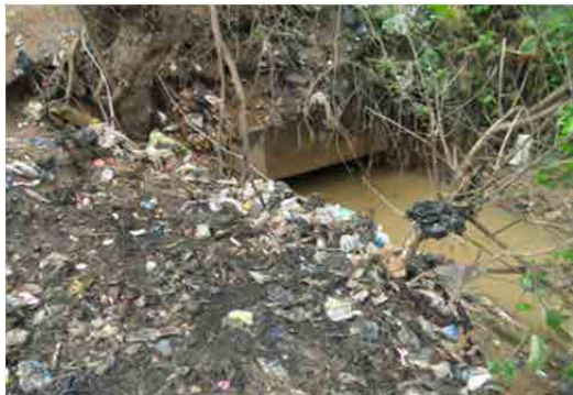
Photo 2.3.32 Culvert Filled with Garbage in Kojokrom Station
