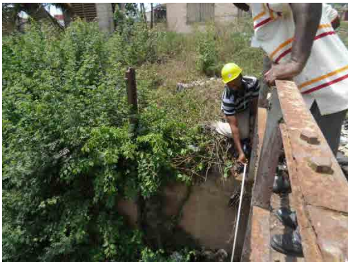
Photo 4.2.22 Measurement of Span Length
