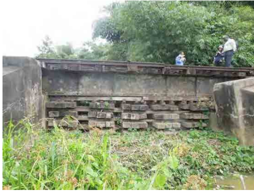
Photo 2.3.34 Steel Girder Bridge Temporarily Supported by Sleepers
