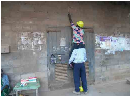
Photo 4.2.46 Hitting Inspection of Shoulders
