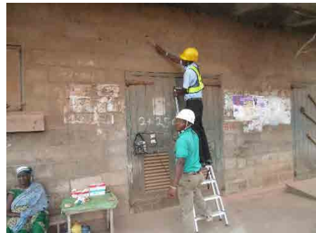
Photo 4.2.47 Hitting Inspection of Concrete on His Concrete by Use a Ladder
