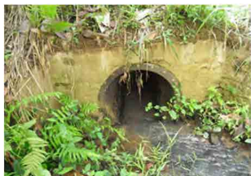
(c) Pipe Culvert (Armco Pipe)
