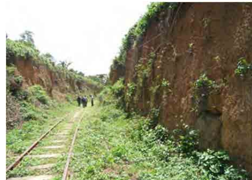
(d) Cut section (laterite soil cut and left as is)
