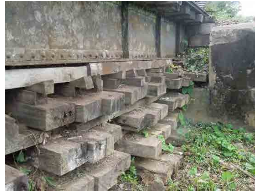
Photo 2.3.34 Steel Girder Bridge Temporarily Supported by Sleepers
