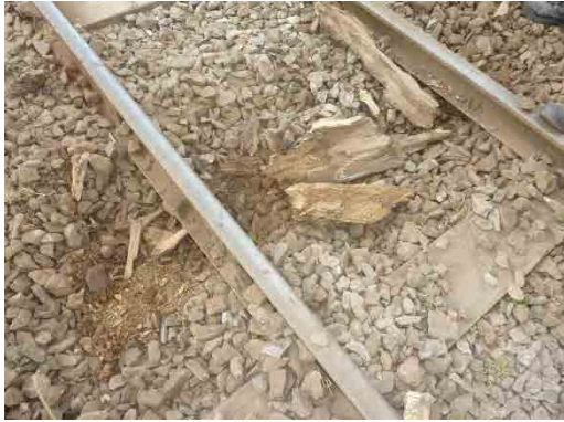
Photo 4.2.62 The rotten sleepers are worn out (This fact means that these sleepers are left as they are rotten for a long time)
