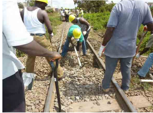
Photo 4.2.63 Trainees are removing the ballast in order to insert the sleeper
