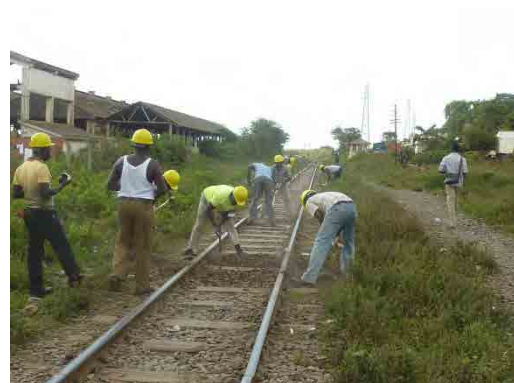
Photo 4.2.61 Every group tried to change rotten sleepers
