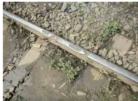
Photo 3.1.12 Trace of the Wheel Slips on the Rail (2)
