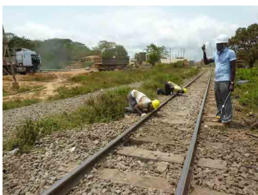
Photo 4.2.70 The Trainees are checking the irregularity of rail low joint
