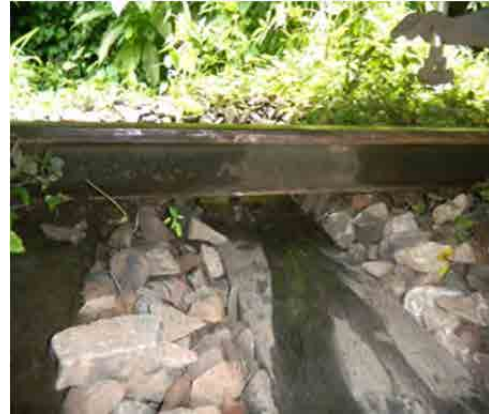
Photo 2.3.20 Trace of Derailment
