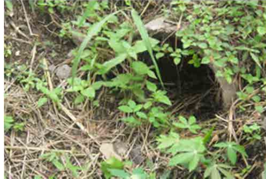
(b) Culvert Covered with the Sediment
