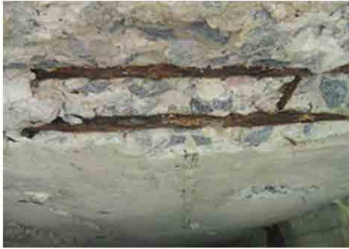
(a) Spalling of the Concrete
