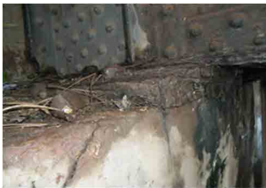
(a) Insufficient Edge Distance (Bridge No.1)
