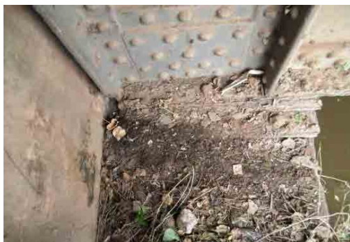
(c) Accumulated Soil around Bearing (Bridge No.1)
