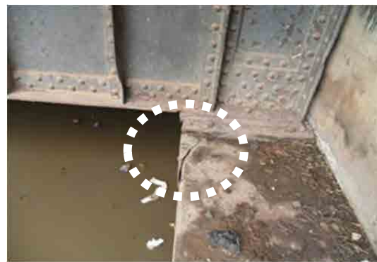
(b) Collapse due to Lack of Edge Distance (Bridge No.1)
