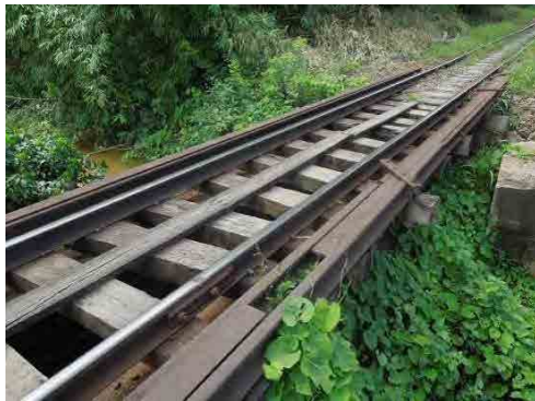
Photo 2.3.36 Track Protection by Rail Girder
