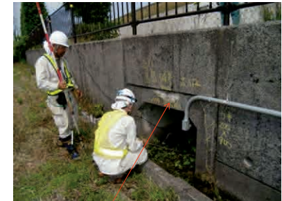
Marking of stripping
