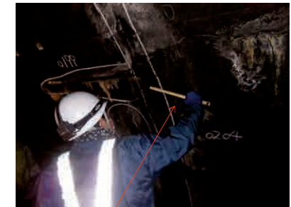
Inspection of float by hammer
