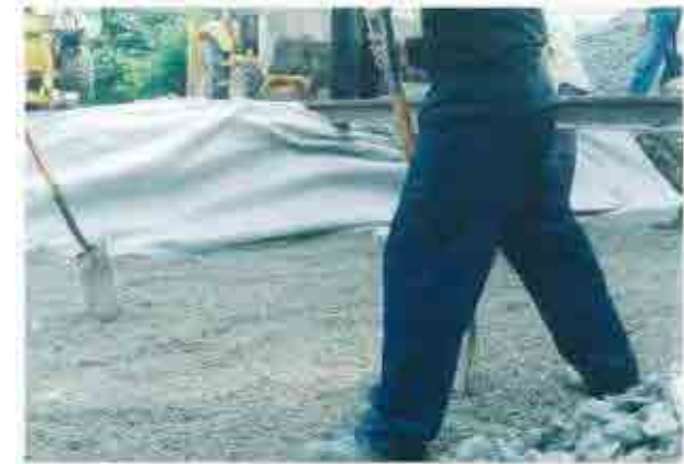
Sand was leveled by the workers. (Example of Thai railways' rehabilitation works )
