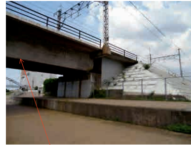
Prestressed concrete girder(5spans)
