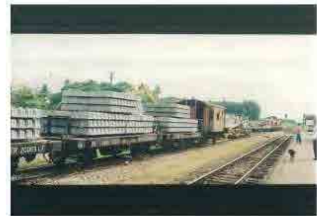
PC sleepers were transported by the trolleys to the site.(Example of Thai railways' rehabilitation works )
