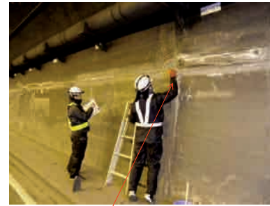
Marking of stripping
