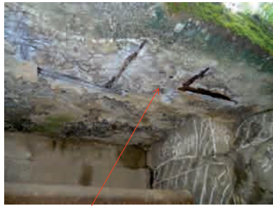
Marking of stripping
