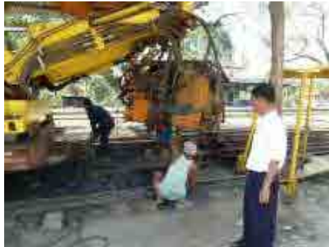
On rail Flash Butt Welding machine
