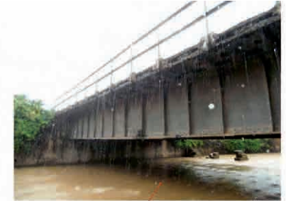
High water level
