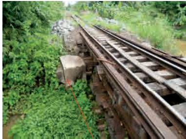
Collapsed abutment
