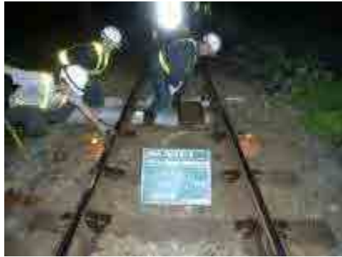
.Installing PC sleeper by man power (Japanese Railway Company)
