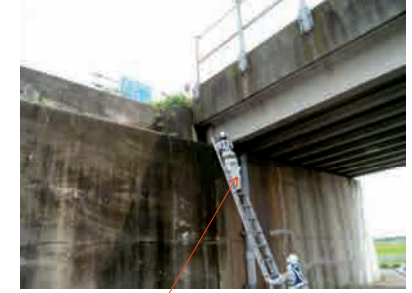
Inspection by ladder
