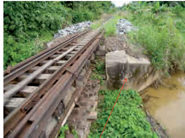
Collapsed abutment
