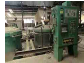
Maintenance facility in an unusable condition
