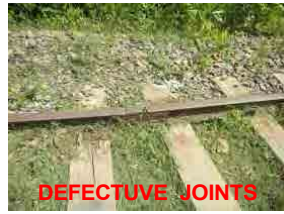
DEFECTIVE JOINTS
