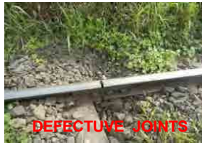
DEFECTIVE JOINTS
