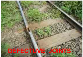
DEFECTIVE JOINTS
