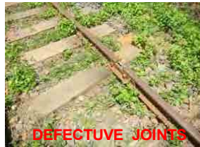
DEFECTIVE JOINTS
