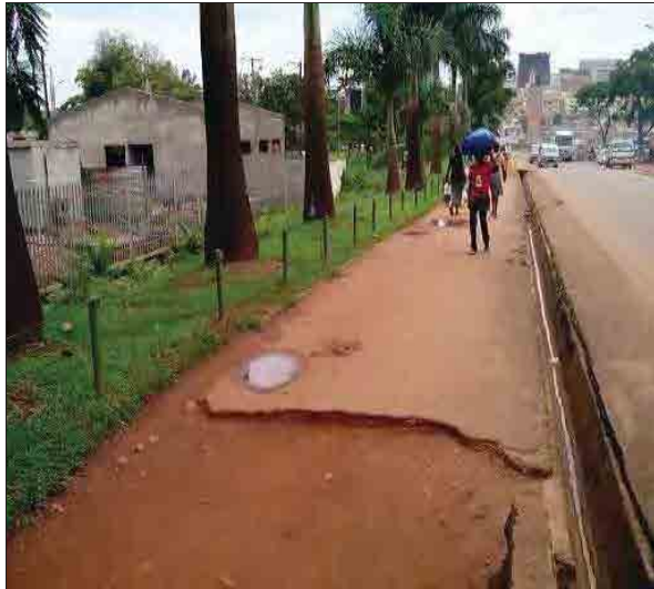
LHS: Existing Queensway Substation CENTRE: Sidewalk with drainage channel RHS: Queensway
