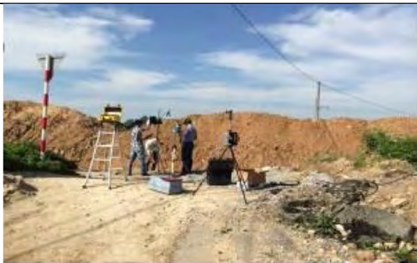
Ph-15 Connecting point with National Route 18 (in QN Province) Noise and vibration measurement
