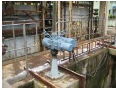
Figure 3.7 Electric motor driven gear actuator
