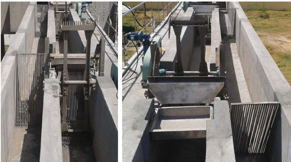
Figure 3.12 UNIDO type arc screen
