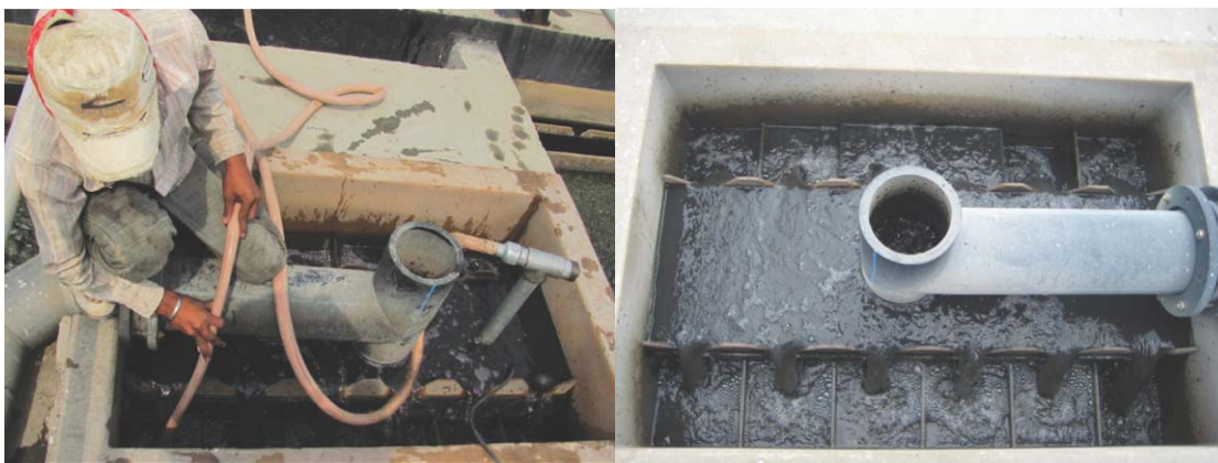
Cleaning of feed pipes by submersible pumps
