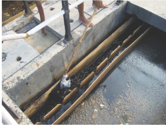
Figure 4.22 Cleaning of effluent gutters
