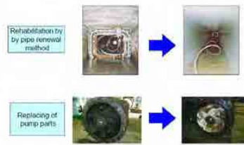
Figure 2 Example of Rehabilitation (SWMD)
