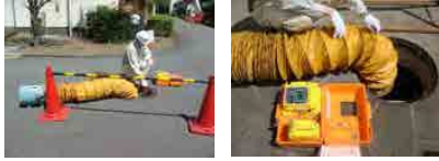
Portable blower and spiral duct
