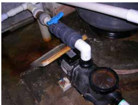
Pic6 Do not remove the plastic cover to protect the pump from drips of seawater.
