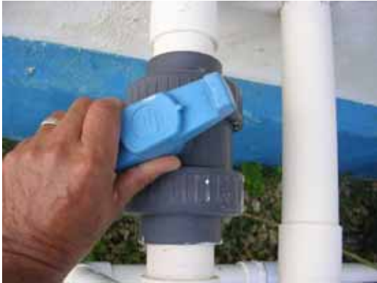
Pic7 Adjust delivery of rearing seawater by seeing water flows at the inlets of the tanks.
