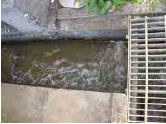
Pic13 Wash the filter material for a while (more than 10 minutes). Discharge muddy water into drainage.
