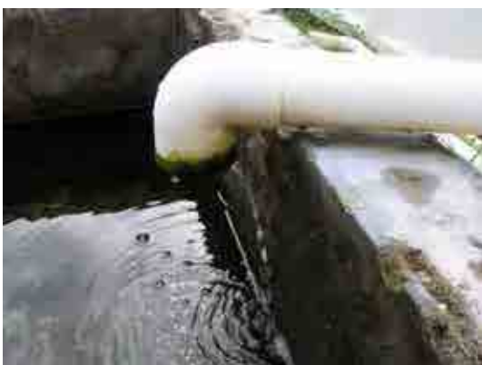
Pic9 For example, seawater can be supplied for more than 3-hours at this flow-rate. If water supplies at the normal flow-rate, the storage tanks become empty within 1 hour.
