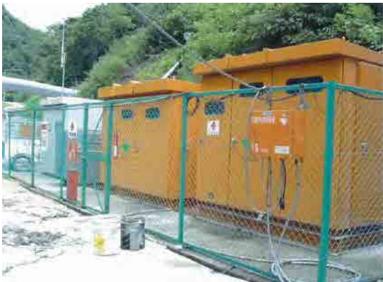
Electric Power Station and Receiving Box
