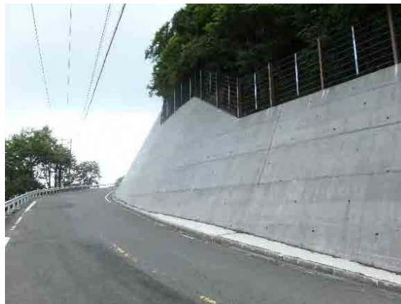
PHOTO 10.2-10 WORKING EXAMPLE OF CONCRETE PITCHING
