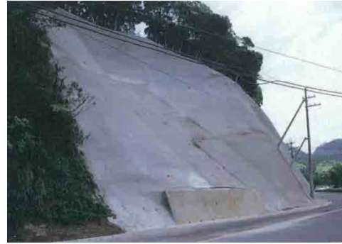
PHOTO 10.2-8 WORKING EXAMPLE OF MORTAR/CONCRETE SPRAYING (SHOTCRETE)
