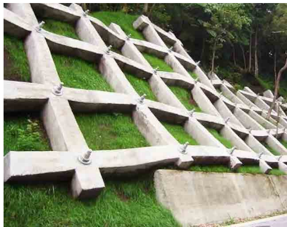
PHOTO 10.2-17 WORKING EXAMPLE OF GROUND ANCHOR (WITH GRATING CRIB WORKS USING SHOTCRETE)
