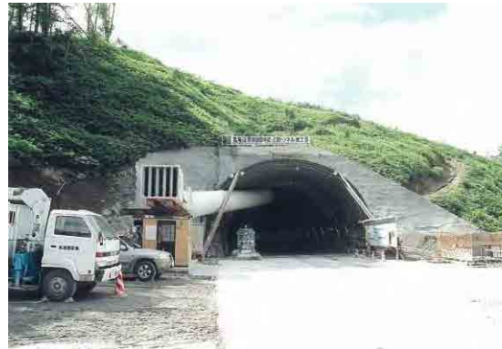
Entrance of Under Construction Tunnel
