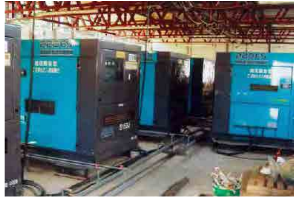
Generator Room for Tunnel Construction
