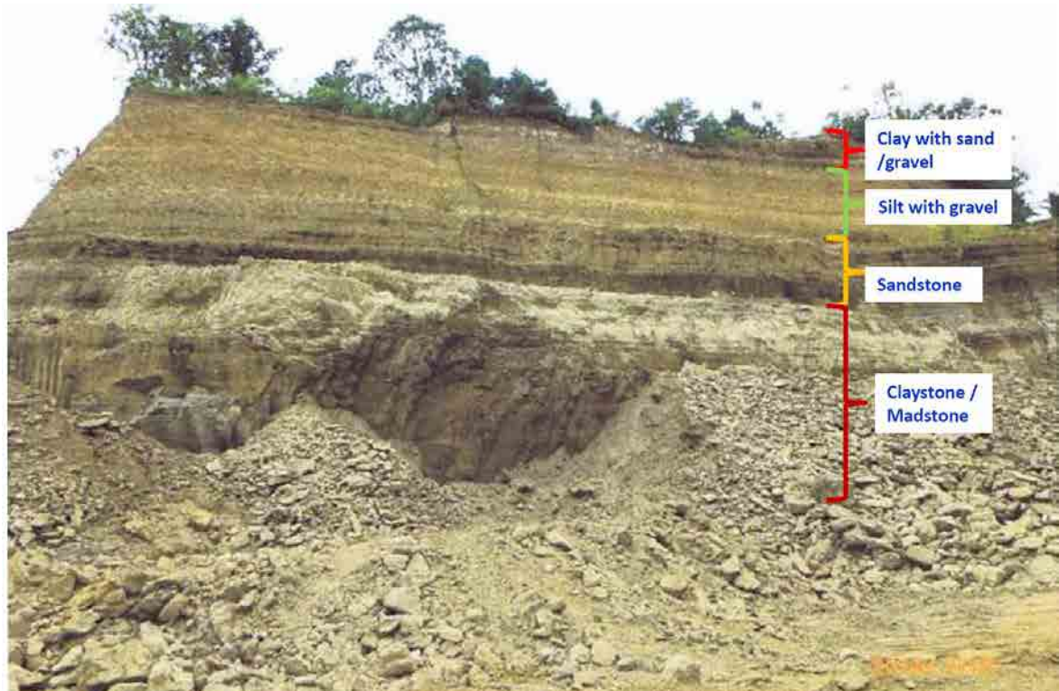
PHOTO 10.4-1 EXCAVATED CONDITION AT QUARRY SITE (ABOUT 1KM AWAY FROM THE TUNNEL SECTION)
