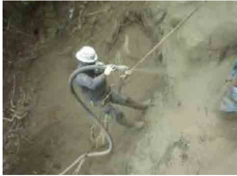
PHOTO 10.2-8 WORKING EXAMPLE OF MORTAR/CONCRETE SPRAYING (SHOTCRETE)
