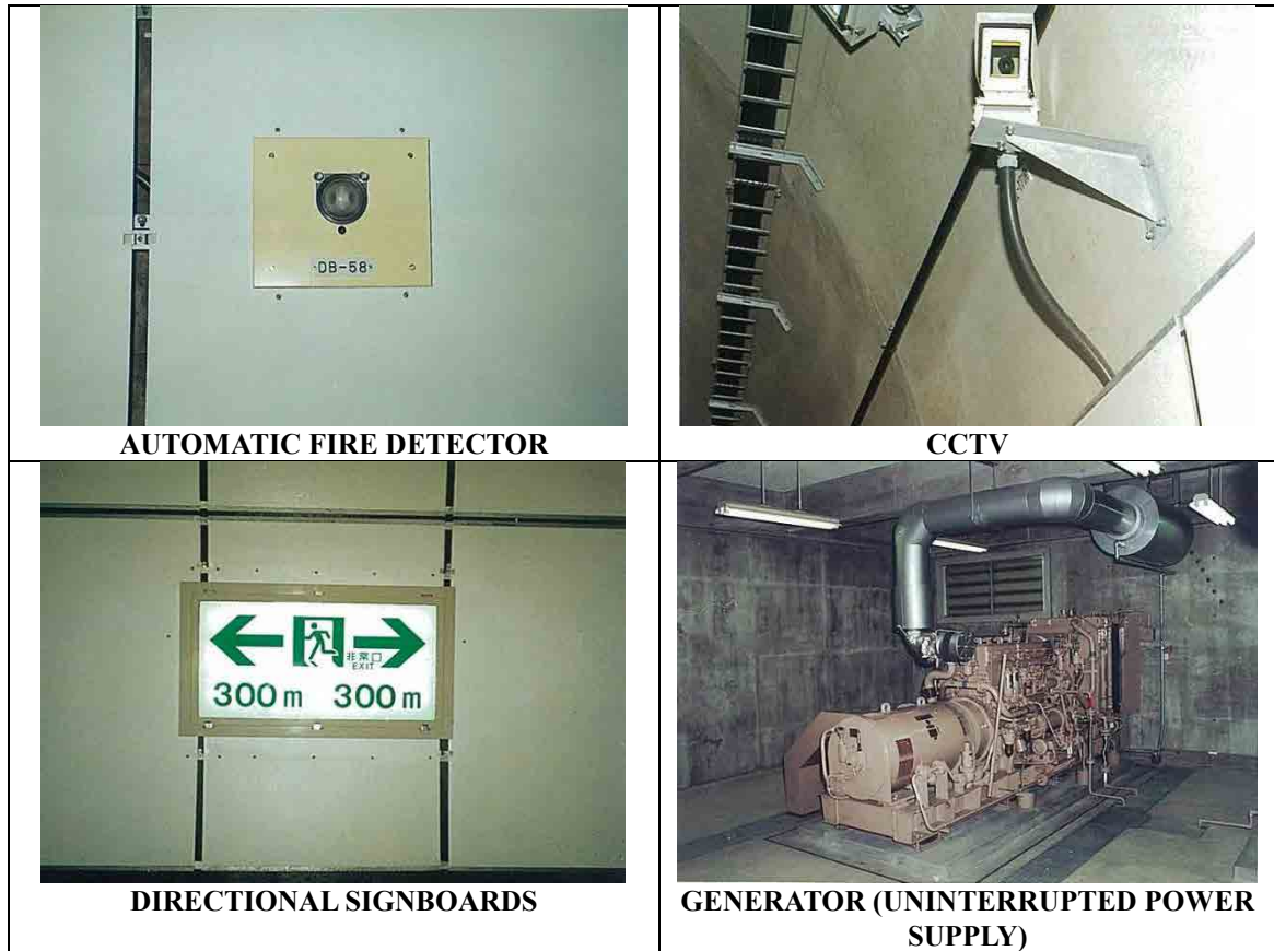
Source: Japan Highway Corporation
