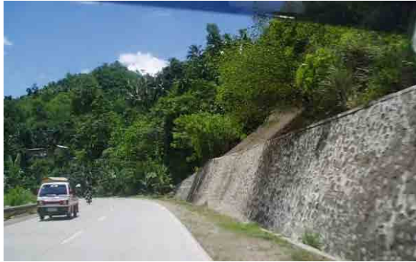
PHOTO 10.2-13 WORKING EXAMPLE OF STONE/RUBBLE-CONCRETE MASONRY
