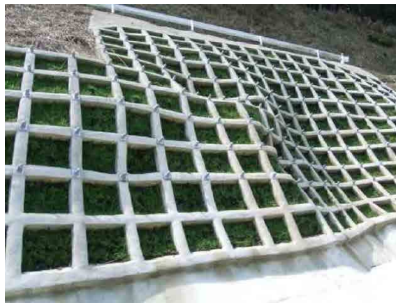
PHOTO 10.2-15 WORKING EXAMPLE OF ROCK BOLT TYPE ANCHOR (WITH GRATING CRIB WORKS USING SHOTCRETE)
