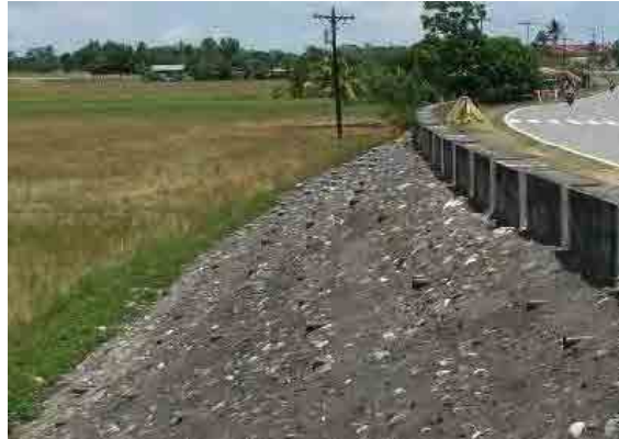
PHOTO 10.2-9 WORKING EXAMPLE OF GROUTED RIPRAP
