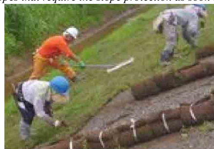
PHOTO 10.2-6 WORKING EXAMPLE OF SODDING
