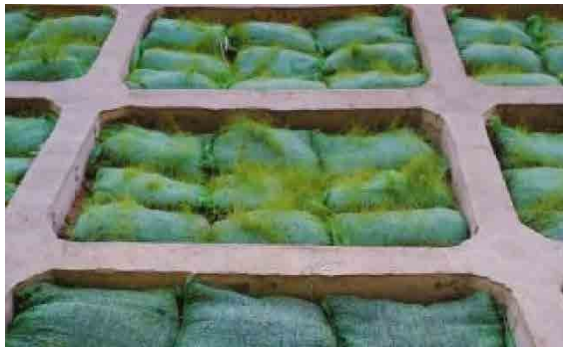
PHOTO 10.2-5 WORKING EXAMPLE OF VEGETATION SANDBAG
