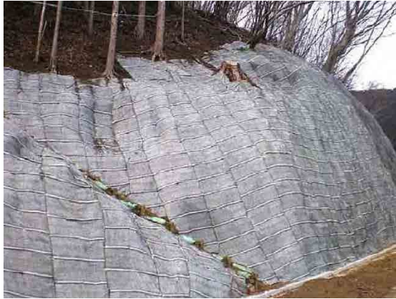
PHOTO 10.2-4 WORKING EXAMPLE OF VEGETATION MAT
