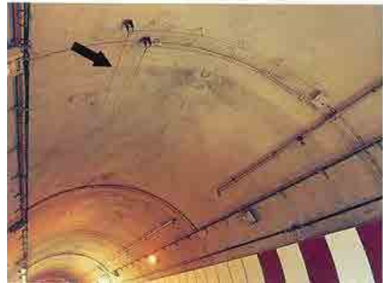
Source: Japan Highway Corporation
