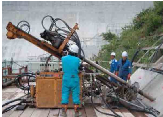
PHOTO 10.2-16 CONSTRUCTION STATUS OF GROUND ANCHOR
