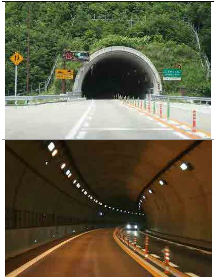
PHOTO 10.2-1 TWO-LANE TUNNEL IN JAPAN
