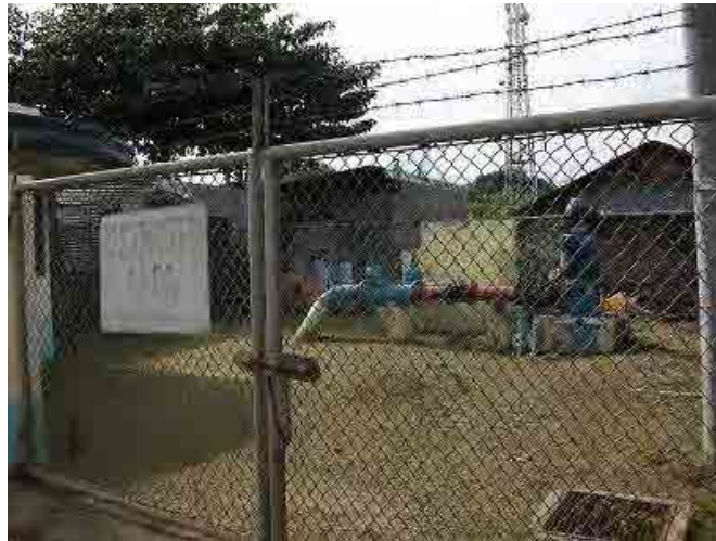
PHOTO 10.1-6 THE WELL OF DUMOY WELL FIELD
