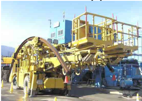
Steel Supports Setting Equipment
