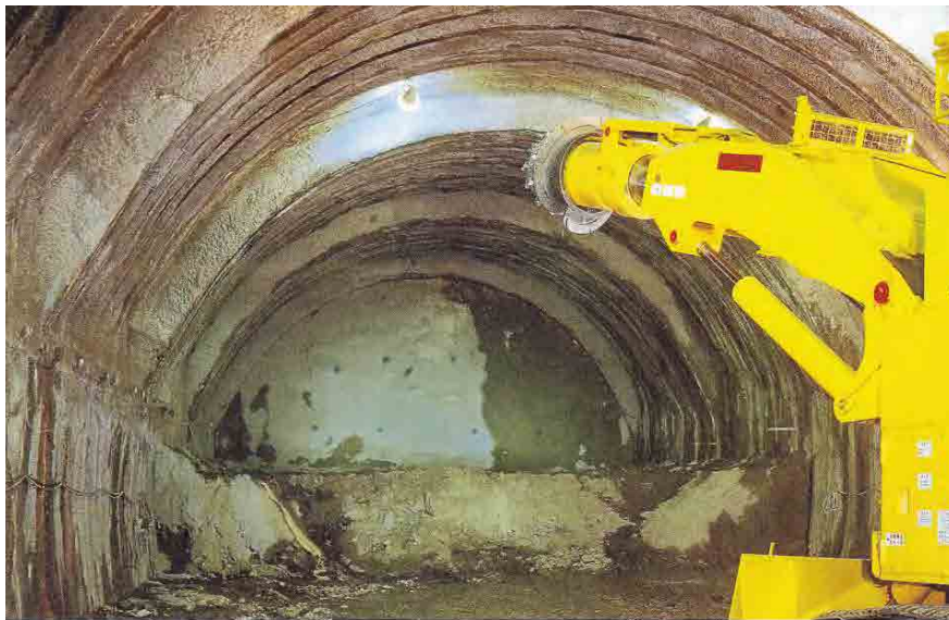
PHOTO 10.4-3 EXCAVATION BY ROOD HEADER
