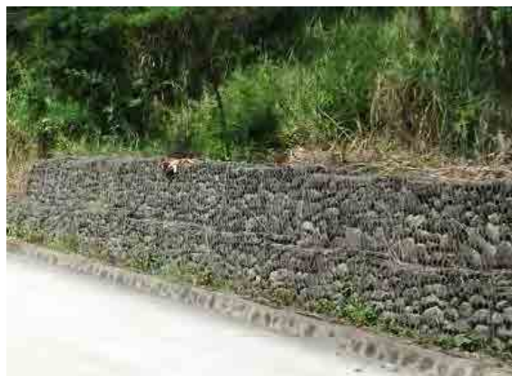
PHOTO 10.2-14 WORKING EXAMPLE OF MAT GABION
