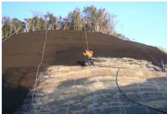
PHOTO 10.2-3 WORKING EXZMPLE OF VEGETATION BASE MATERIAL SPRAYING
