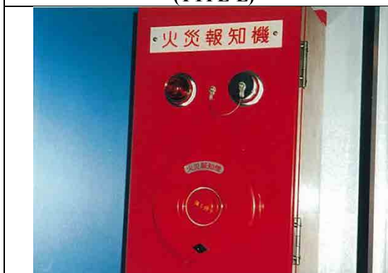
PUSH-BUTTON NOTIFICATION EQUIPMENT
