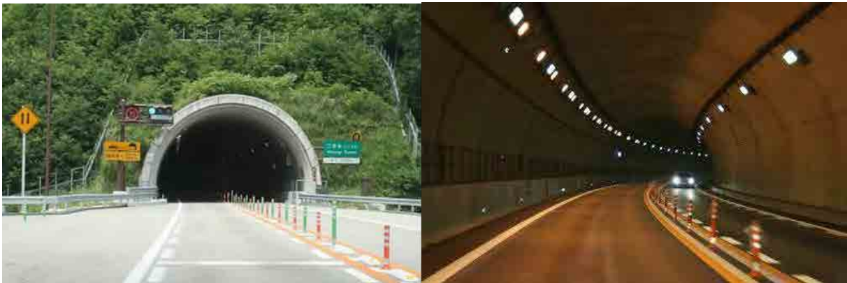
Two-lane Tunnel in Japan
