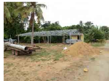
Construction of hatchery Farmer A (Mr. Prum Vat)
