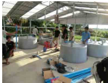
Installation of tanks Farmer B (Mr. Hang Heang)
