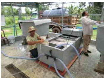
Plumbing the filter tank Farmer C (Mr. Van Po)
