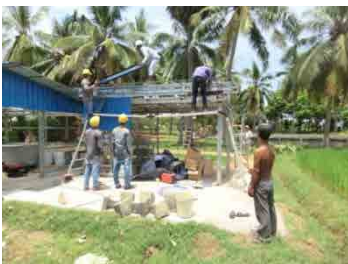
Installation of solar panel Farmer C (Mr. Van Po)
