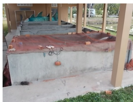
Pic. 14. Rectangular tank (4x1.8m).
