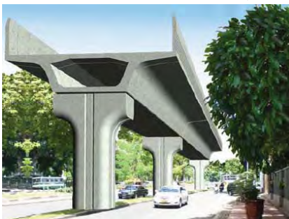
Elevated Guide way
