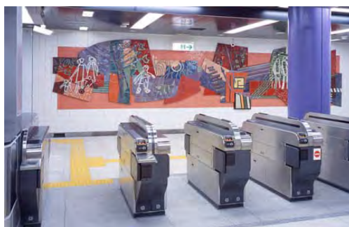
Photo 3.9-1 an AFC Gate (Toei Oedo Line, Tokyo, Japan)
