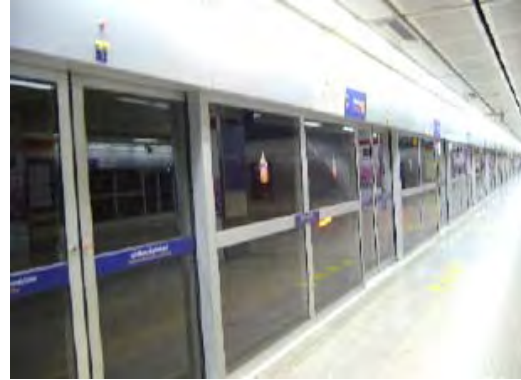
Full-height type in Bangkok (underground station)
