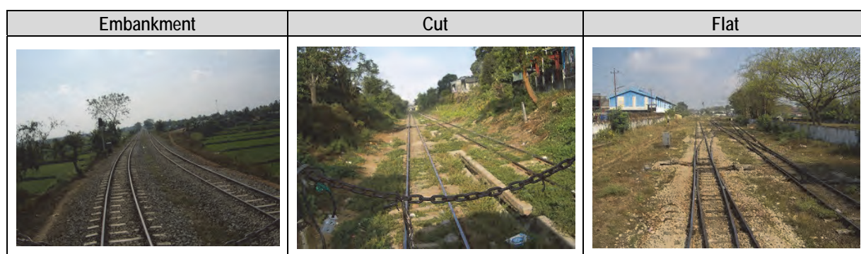
Figure 3.1.2.1 Typical Condition of Embankment, Cut and Flat Section
