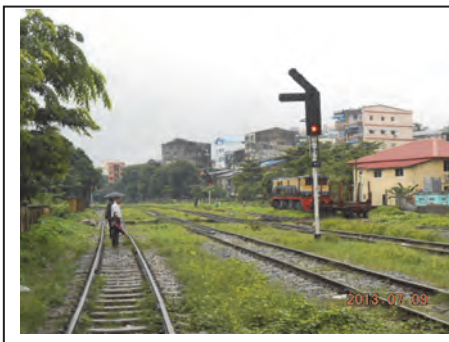
Figure 3.3.1.1 Current Automatic Block Colour Light Signal
