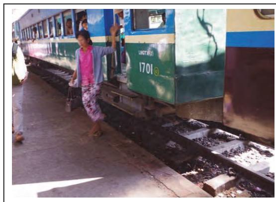
Figure 3.4.1.2 Low Height Platform
