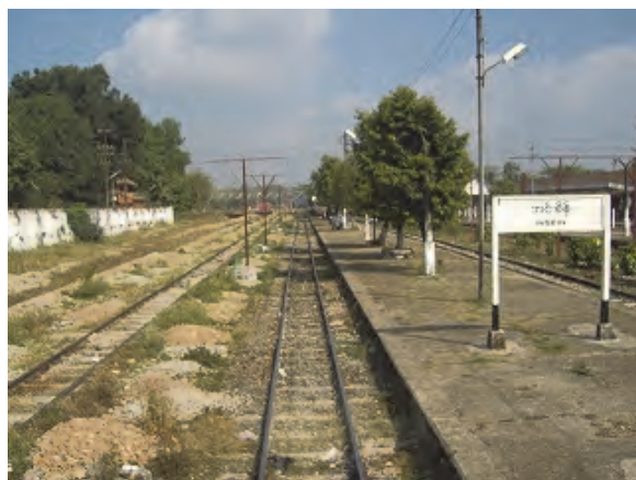
Preparing the ballast along platform
