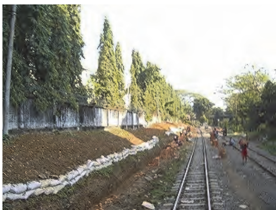
Under construction retaining wall
