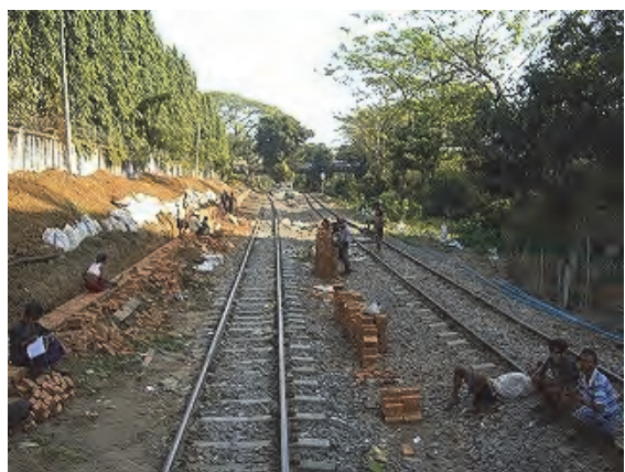
Under construction retaining wall
