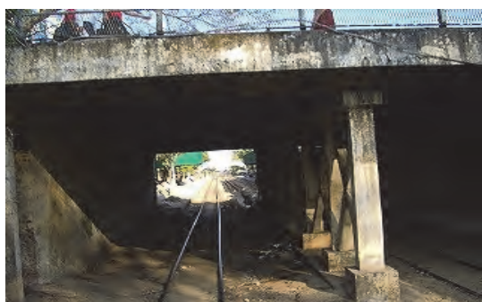
Passing under the ROB (Not enough height for electrification)
